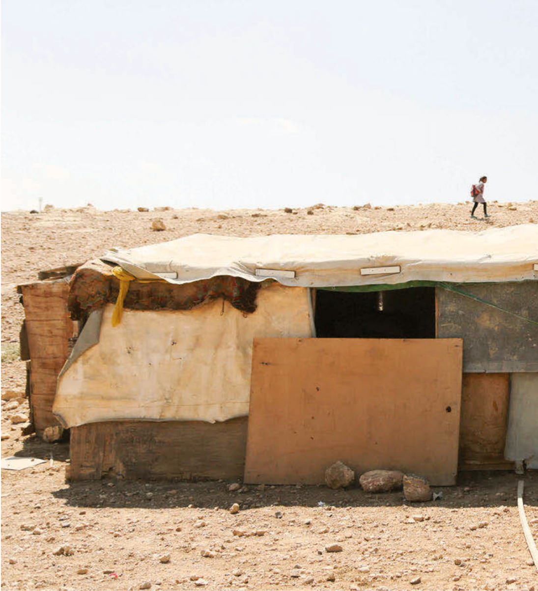
▲ Jahalin Construction, Khan Al-Ahmar, 2014.
