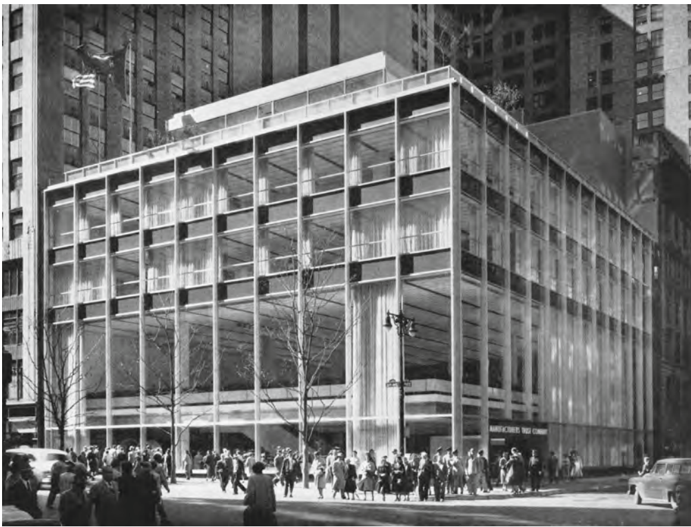
4 Former Manufacturers Trust Company Building, New York, USA, 1953–1954, Skidmore, Owings & Merrill (SOM)/Gordon Bunshaft.
