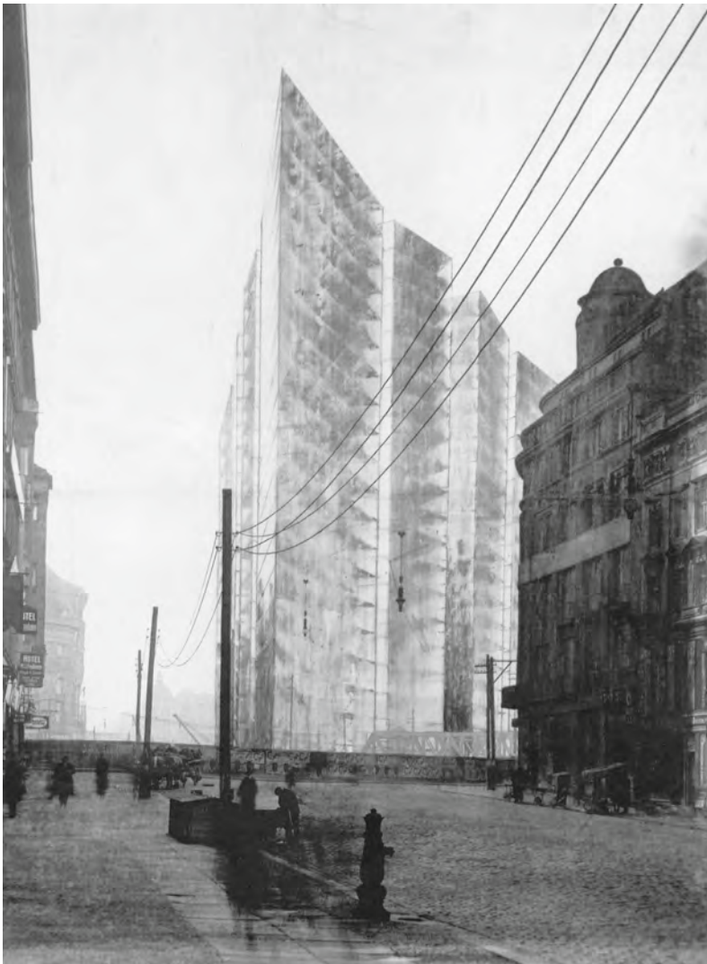
1 Design for a high-rise building on Friedrichstrasse, Berlin, Germany, photomontage, 1921, Mies van der Rohe.
