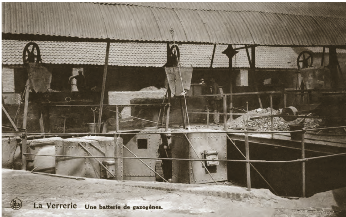
3 Battery of gas producers for a tank furnace, late 19th or early 20th century, Belgium, photographer unknown.
