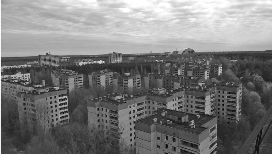
Figure 5.1 Panorama of Pripyat from the roof of a 16-storey residential tower.
