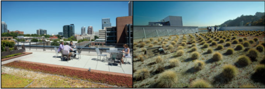
Fig. 18.1 Vegetated ecoroofs, also called green roofs. These features reduce stormwater runoff and pollution and provide wildlife habitat (Source: Portland State University)
