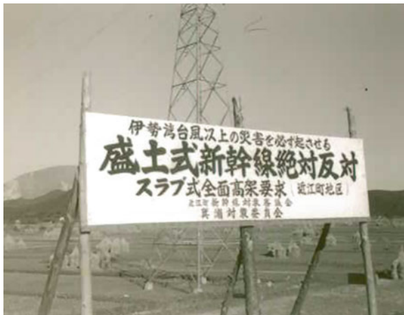
Photo 4.1 A sign opposing the embankment-type Shinkansen. (Source: Shiga Prefectural Government)
