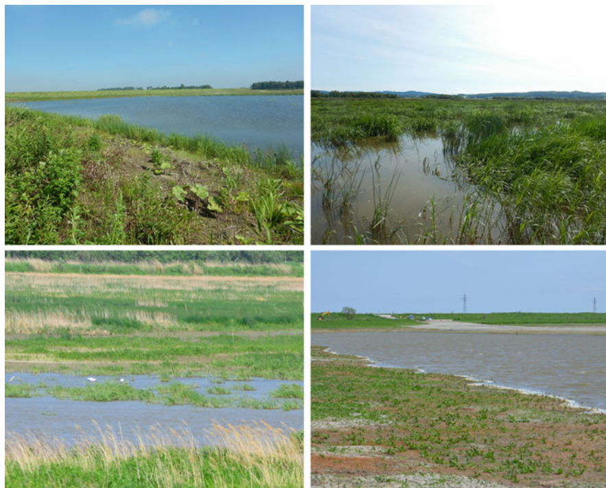
Fig. 12.5 Chitose flood-control basins
