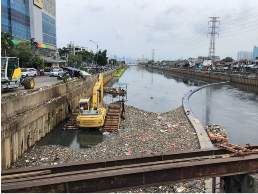
Fig. 21.4 River cleaning activities by local government in Western Banjir Canal (downstream of the Ciliwung river) near the Seasons City Trade Mall (taken by the author on November 30, 2019)
