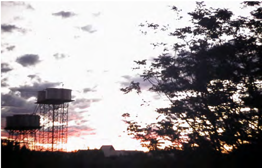
Figure 4.3 The Yuendumu water towers
