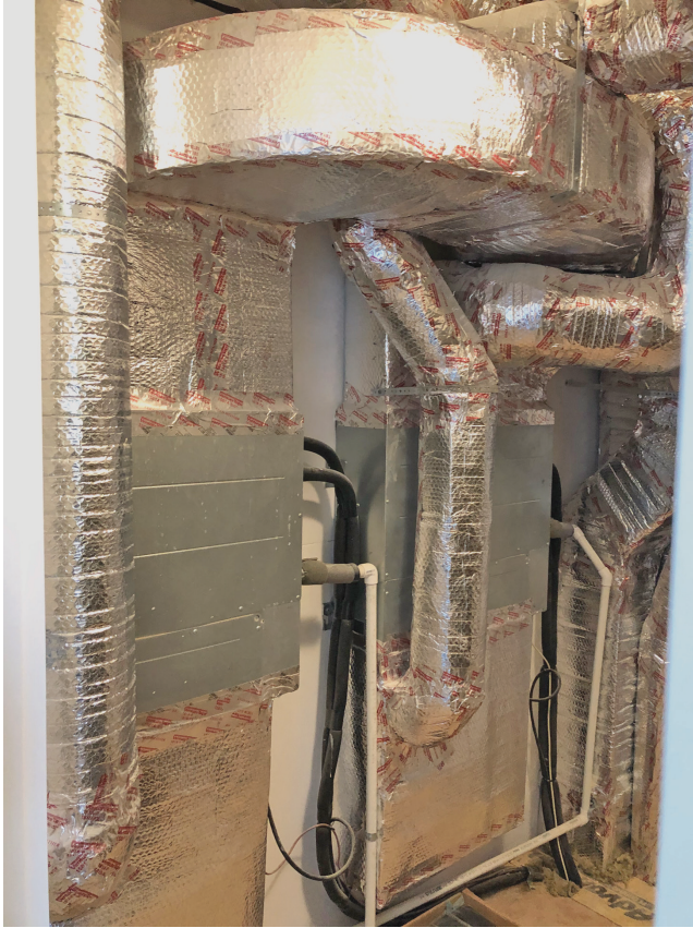
Figure 11.9 Well insulated and sealed ductwork performs better, ensuring comfortable air distribution throughout the whole building.
