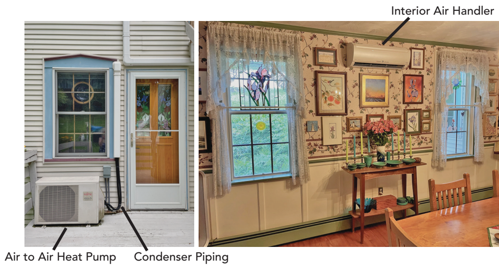
Figure 11.4 Mini split heat pump has a small exterior heat pump unit and a fan coil on the interior.
