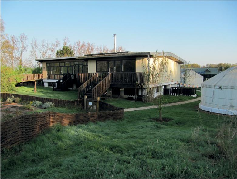
**Figure 9.4** The Solar Building at Othona, made out of compacted clay dug from the ground below and elevated above flood level. Ken Worpole.
