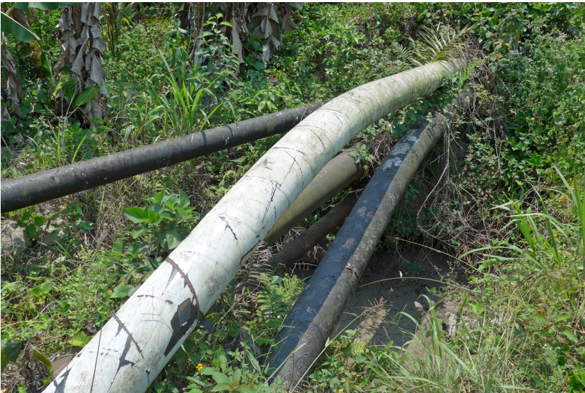
Figure 4.4. Pipelines protruding in a field in Emiliano Zapata, Papantla, Mexico, 2017 © Svenja Schöneich.
