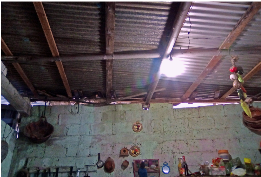
Figure 4.7. Decommissioned pipelines used as ceiling joists of a house in Emiliano Zapata, Papantla, Mexico, 2018 © Svenja Schöneich.
