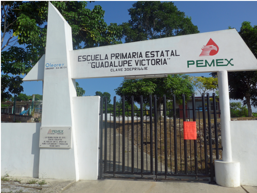
Figure 5.2. Entrance of the primary school renovated by PEMEX and Oleorey in Emiliano Zapata, Papantla, Mexico, 2016 © Svenja Schöneich.
