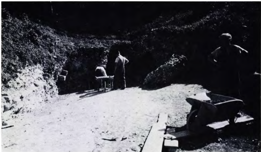
b. Work on the barrel vault between 12c and 12d The cellars
