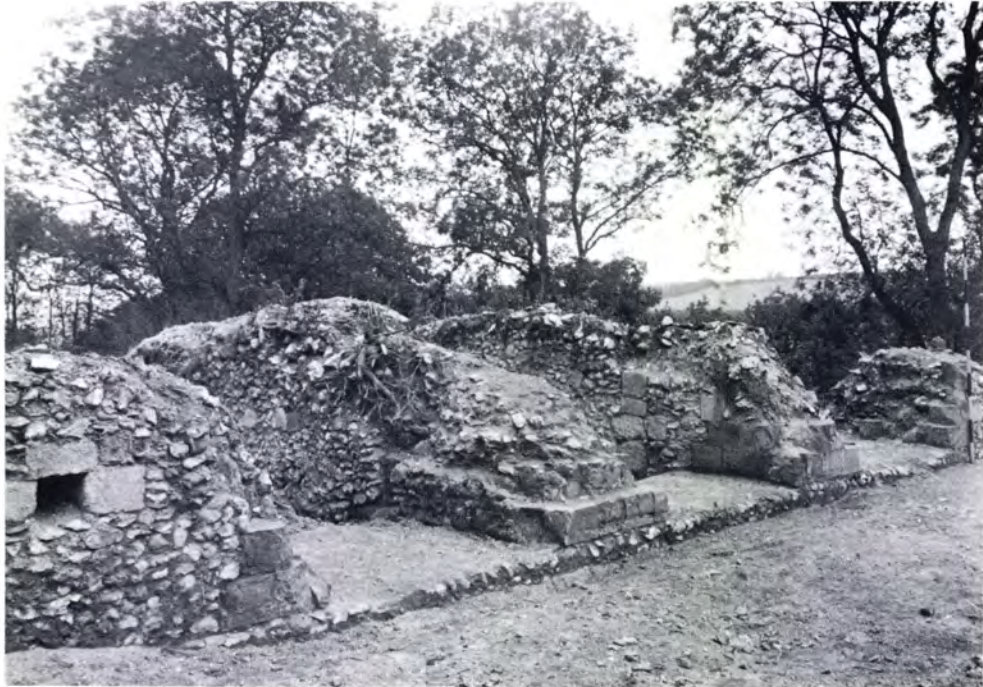
a. The three entrances from the great hall (5) into the servery/buttery rooms (4b and 4c)
