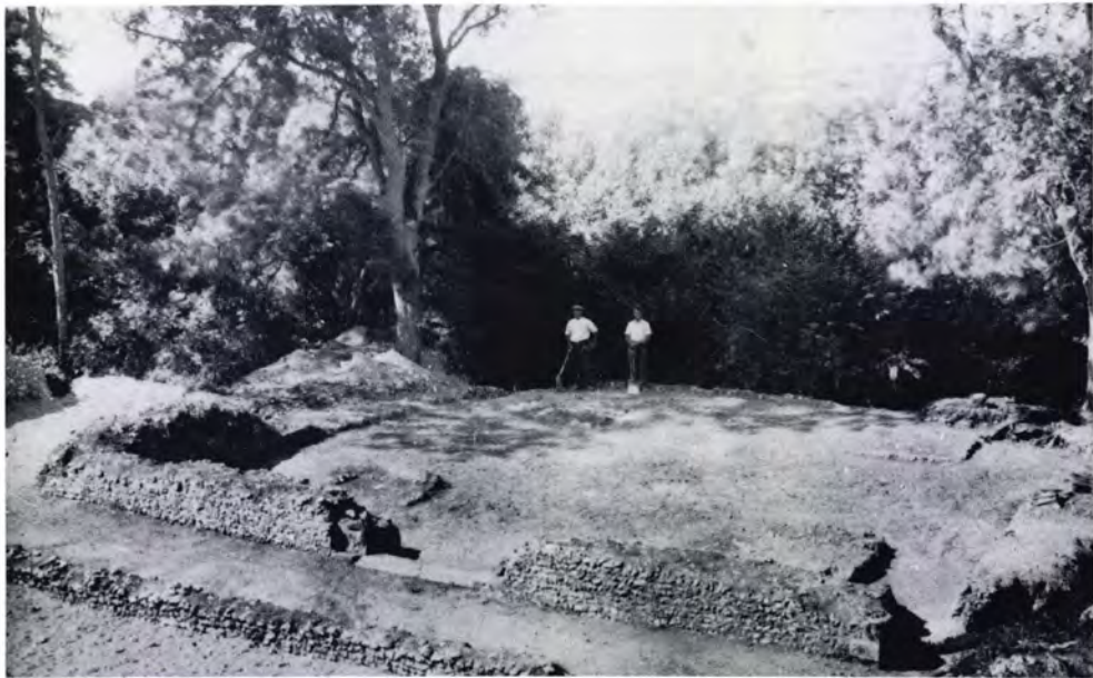
b. The north kitchen (4e), looking north. The four pillar bases can be seen, and also the wide chamfer of the threshold
