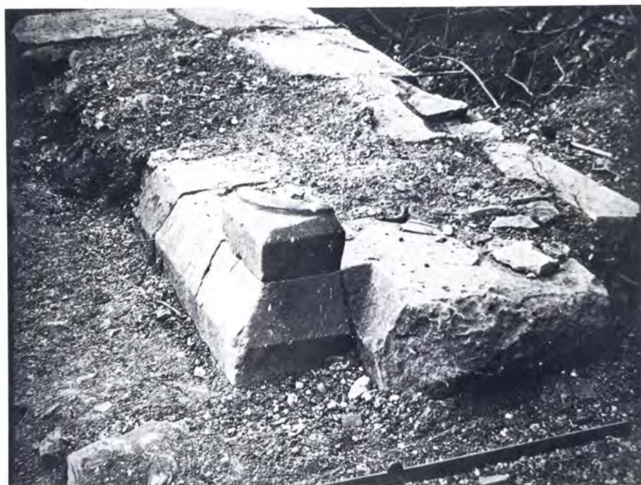
b. The south porch ( 5b ), looking south-east from inside, showing the chamfered plinth and column base. The double skin and core filling construction is clearly seen
