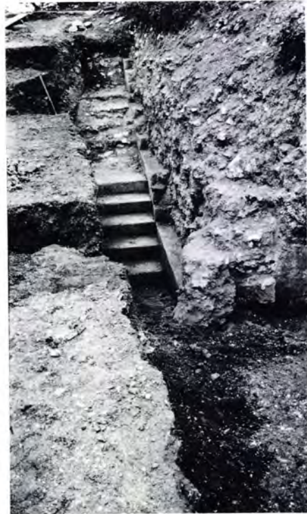
c. Trenching the east side of the cellar stair ( 12b ), 26 September 1938
