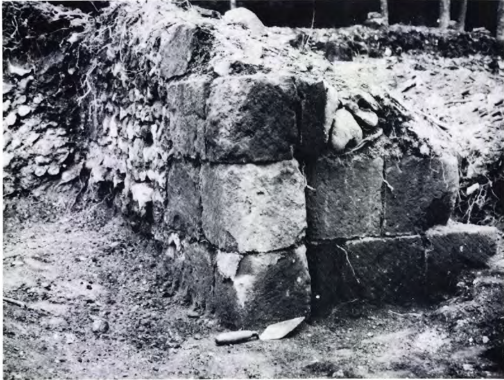
a. Ashlar entrance to the west kitchen ( 4h ), looking south-west. The rebate is formed by projecting blocks of masonry. Diagonal tooling is clearly visible
