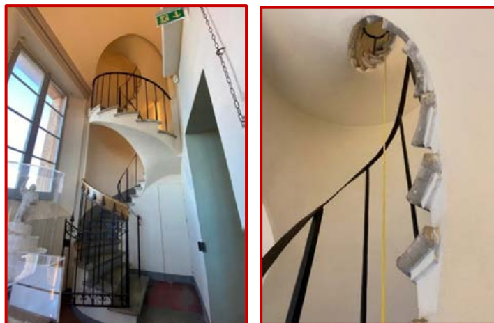
Fig. 3: Spiral staircase from the 4th to the 7th floor of the tower
