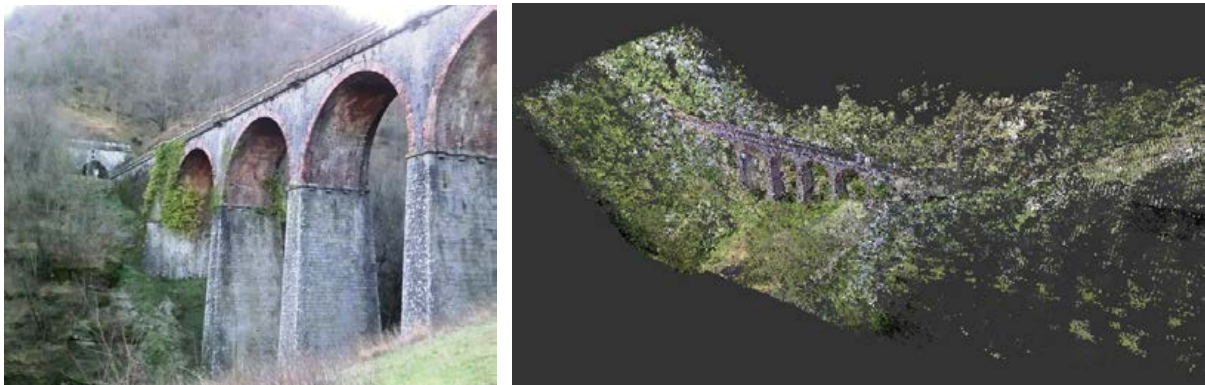
Fig. 1, 2: Masonry bridge over Masera Ditch | Laser scanner survey.
