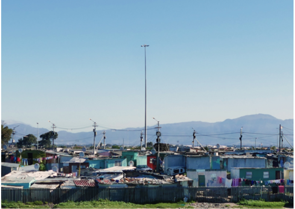
Fig 12 Barcelona Informal Settlement in Khayelitsha, with the two lighting solutions – lights on electricity distribution poles and high-mast lighting
