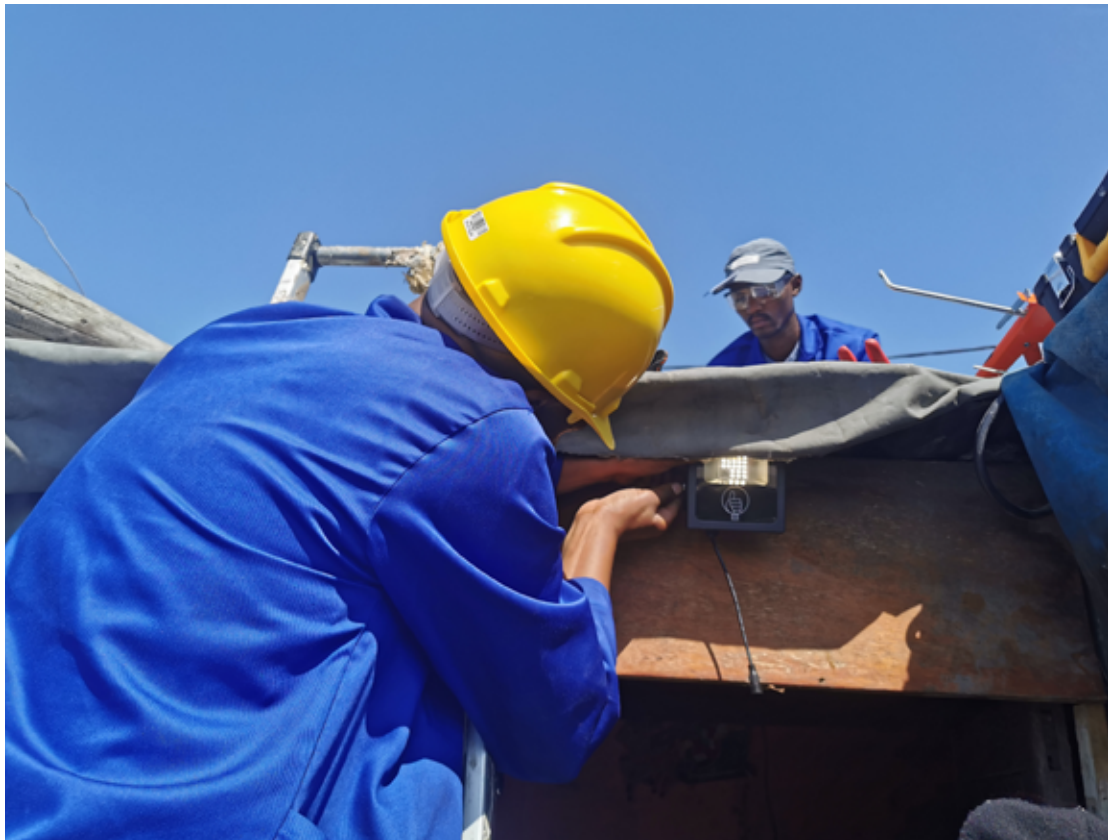
Fig 4 Installation team installing a wall-mounted solar light
