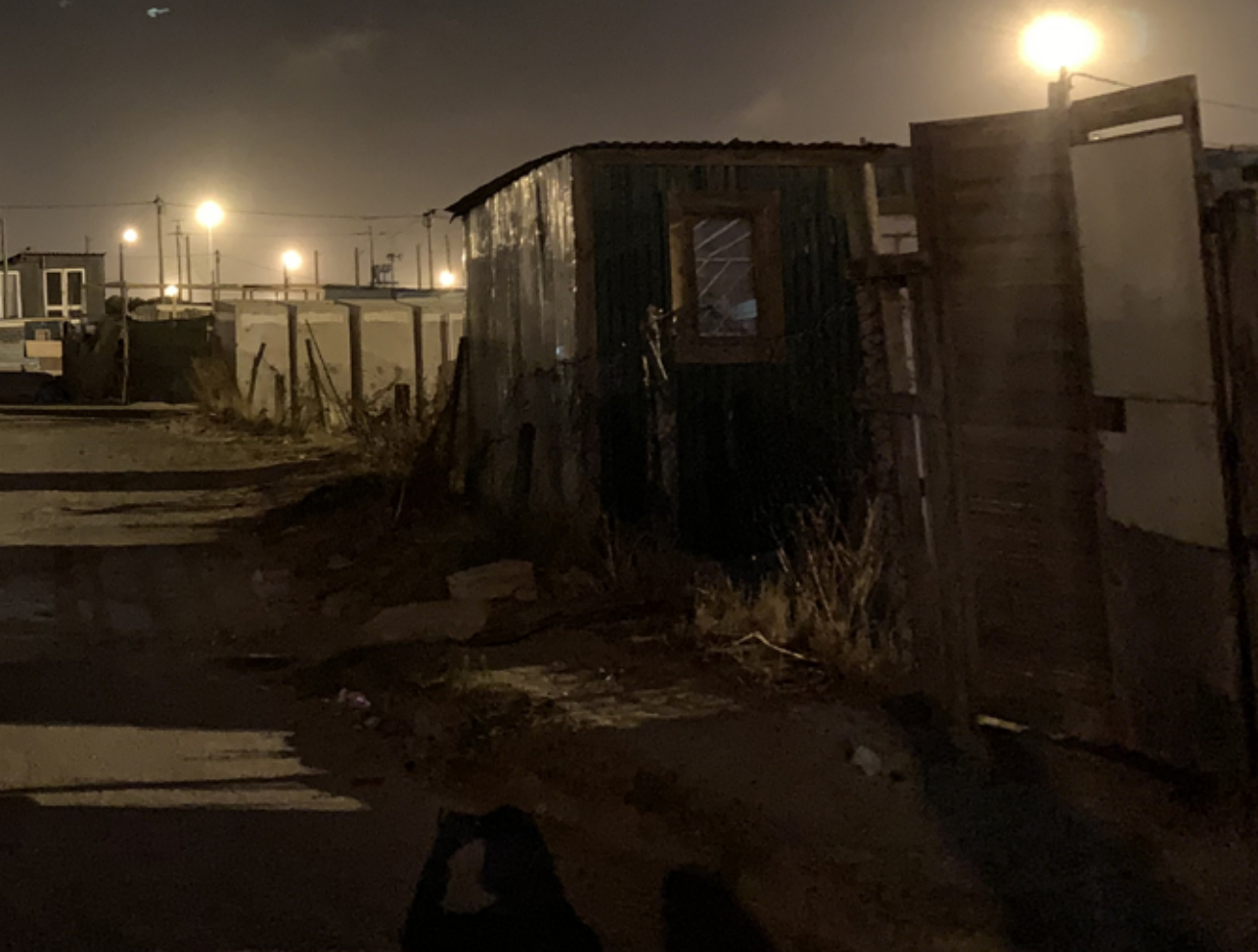
Fig 6 Neighbourhood-scale view of high-mast lighting in SST Informal Settlement
