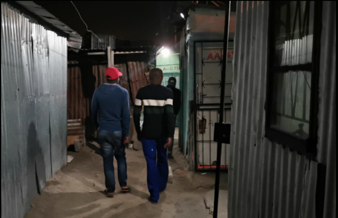
Fig 9 Brightly lit pathway after installing new solar public lights in PJS
