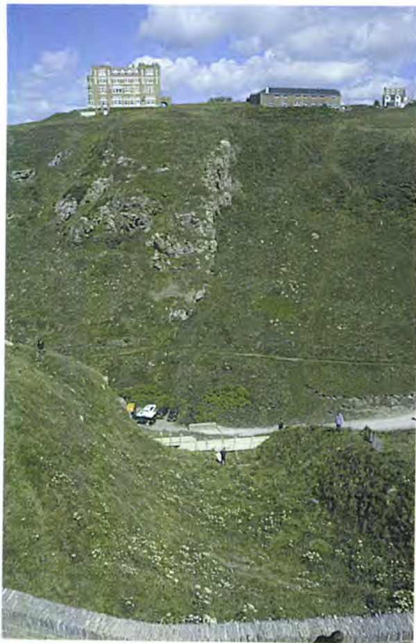
90 Geological fault on the east side of the valley, from the west.
