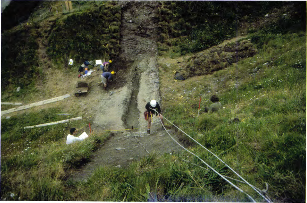
95 Photograph of Vertical Technology and planning T01. Photograph: K J Brady
