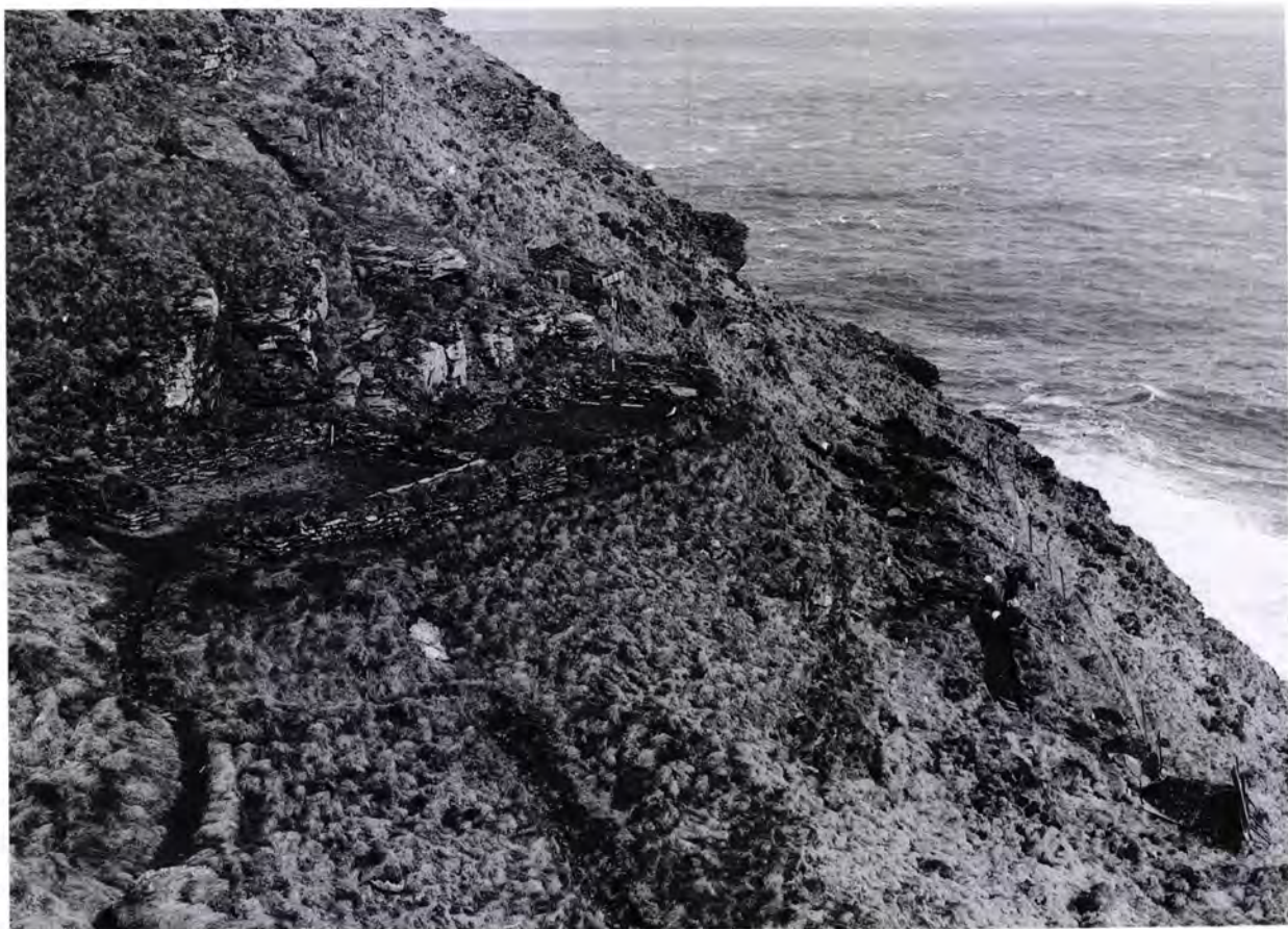
27 Work on the Lower Terrace area excavation in 1991, viewed from the southern end of the terrace. Photograph: C D Morris (Harry and Morris 1997)
