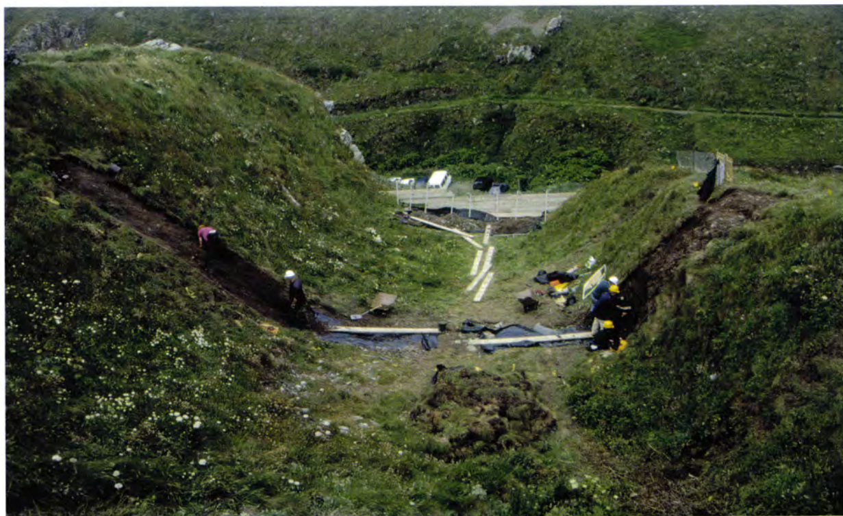
94 Excavation of trench T01. Photograph: K J Brady
