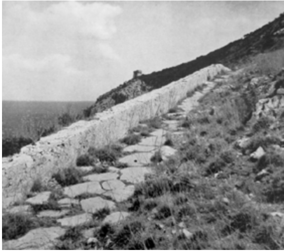
Fig. 2. Massa Lubrense, Punta Campanella. The ancient paving of via Minervia characterized by a halfway up the hill path [PANE 1955, p. 45].
