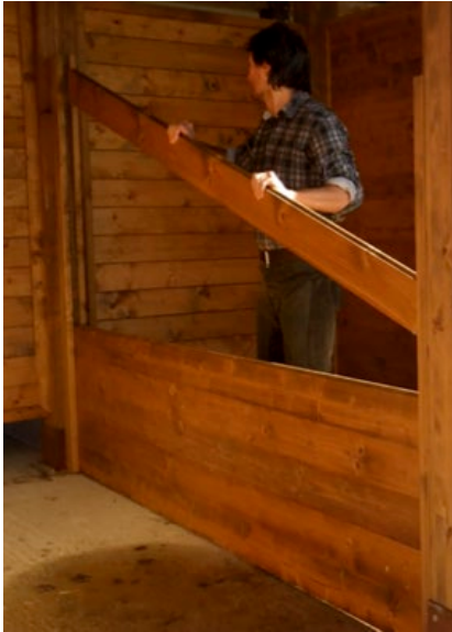
Fig. 7. Particular of innovative type of horse shelter
