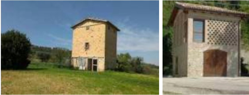
Fig. 4.1 Dryer “F” with adjacent courtyard (left). Example of a refurbished dryer (right).
