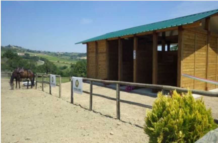
Fig. 6. Structure completed and inaugurated in June 2014
