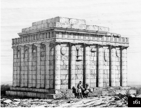
Left 161: Suweida, Tomb of Hamrath, in a print by De Vogüé, 1865; this was much deteriorated by 1909, some blocks being used to build a barracks. Centre, 162: Suweida, temple, photo of 1909. The town “contains about 200 families, of whom 30 are Christians, and all the rest Druses, there being no Mohammedans settled here” (Buckingham, 1825).
