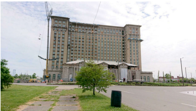
Fig. 12: Michigan Central Station under Reconstruction, courtesy of Juliane Borosch
