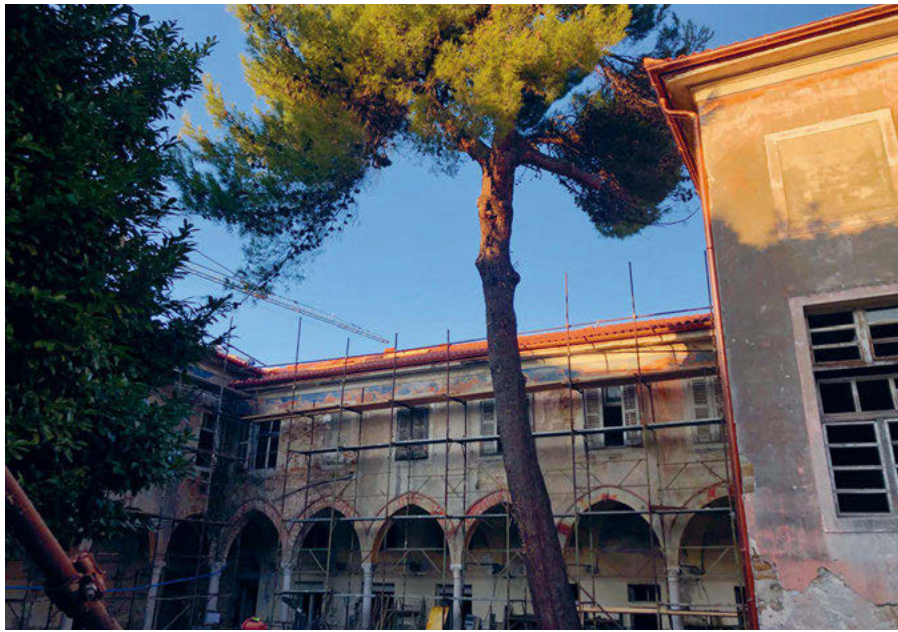
Fig. 4.4 Koper's Servite Monastery 1 courtyard view, Slovenia
