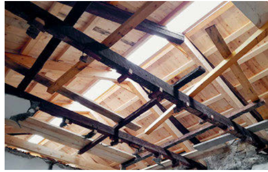
Fig. 4.5 Koper's Servite Monastery ceiling renovation, Slovenia
