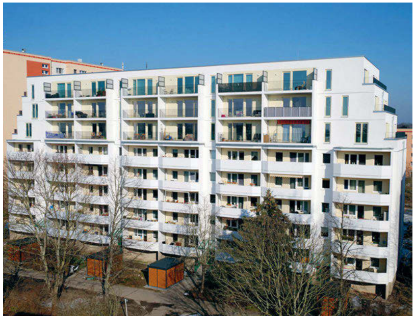
Fig. 11.2 Three-floor extension on a WBS 70, 3 prefabricated building in timber hybrid construction, Berlin
