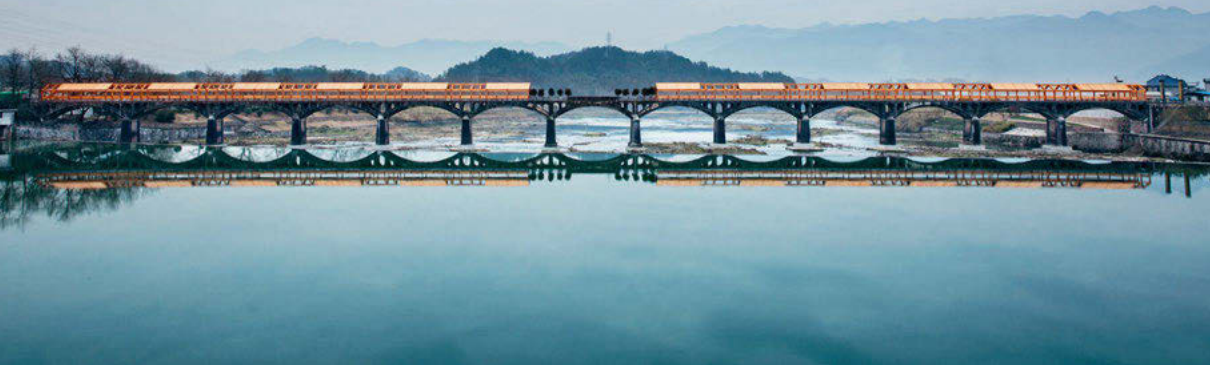
Fig. 5.4 Shimen bridge and river
