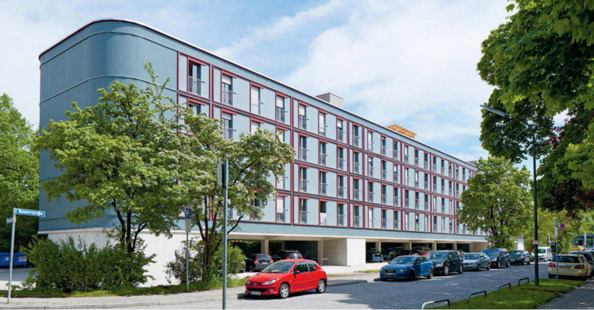
Fig. 11.1 Parking lot superstructure with a timber hybrid building, Dantebad, Munich
