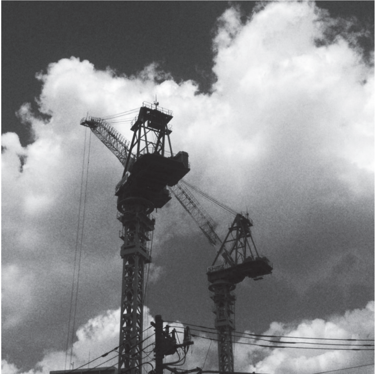
Construction Time Again
