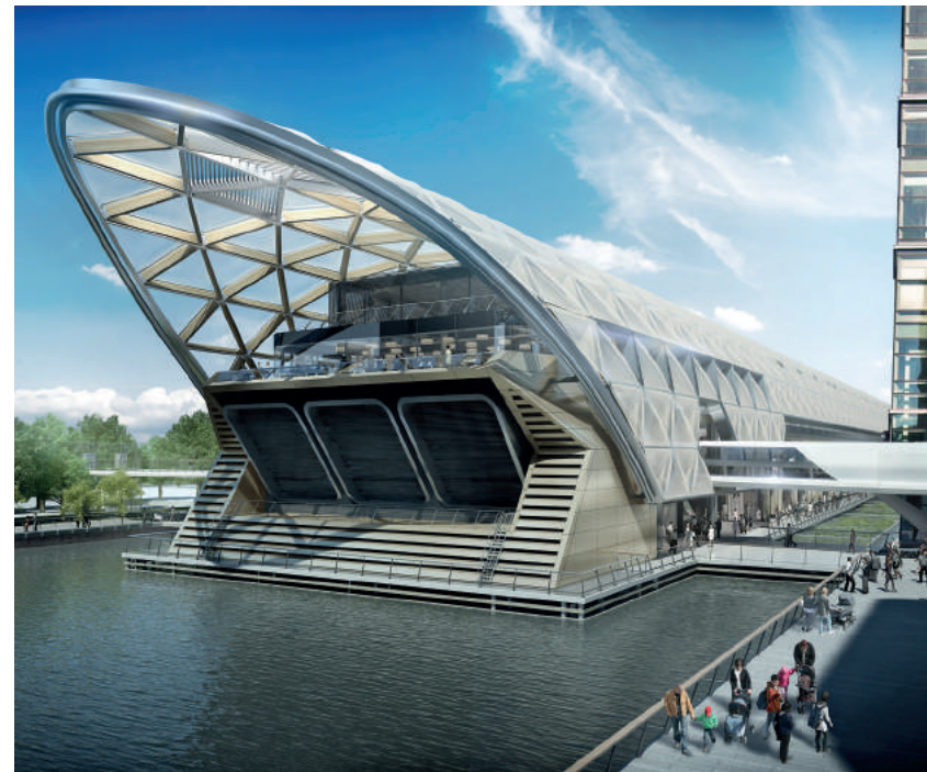
Fig. 2: Rendering showing Foster + Partners design for roof enclosure cantilevering out over the water of the North Dock, Canary Wharf. (Photo: Methanoia / Foster + Partners.)
