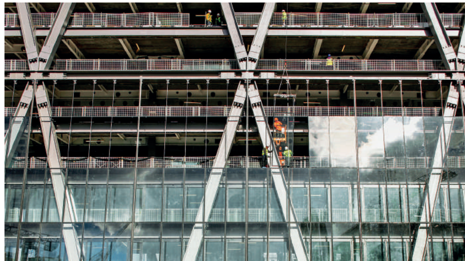
Fig. 7: Node type 7 assembled and forming part of the inclined south face.
