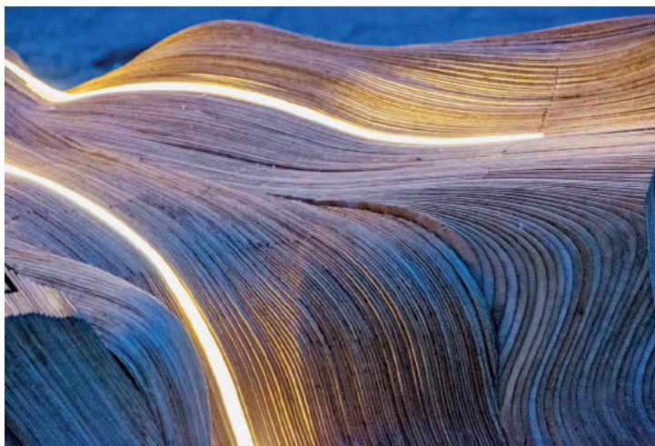
Fig. 12: Detail of integration of luminous LED strips within grain of trunk base.
