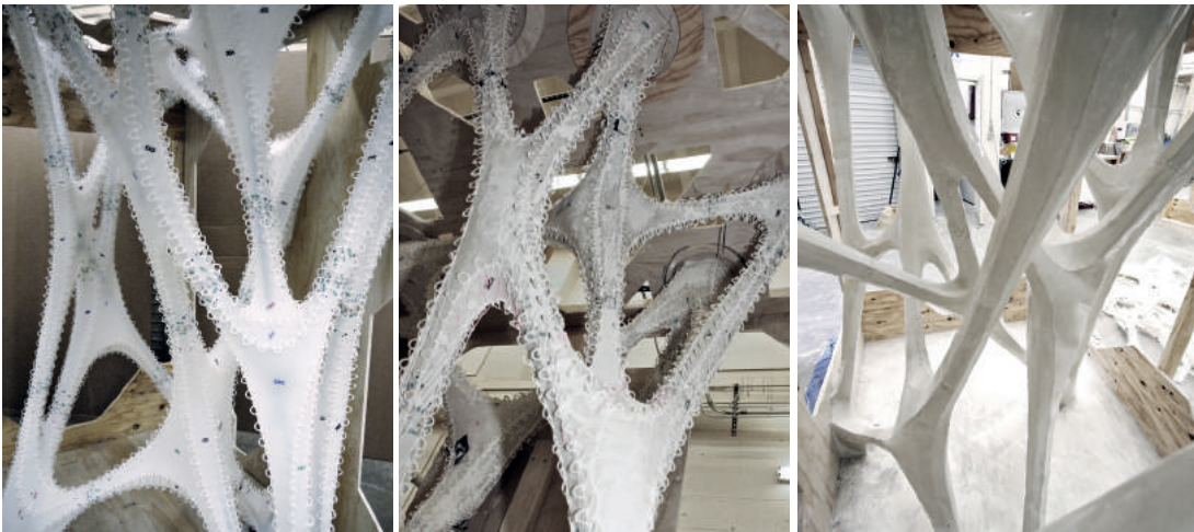
Fig. 12: Casting process: assembled polypropylene formwork, formwork after casting, and unwrapped concrete. (Photos: Craig Gillam.)
