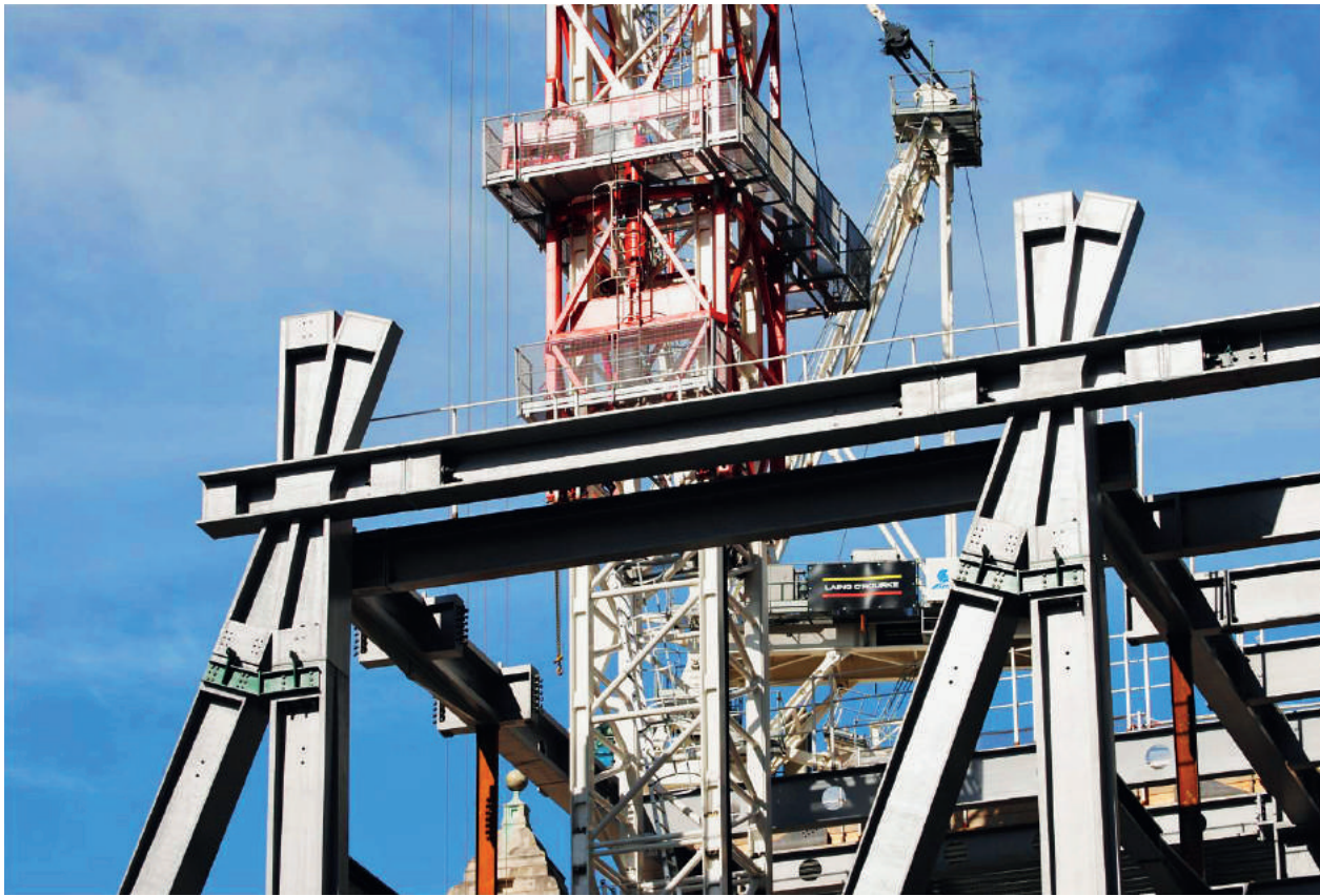
Fig. 14: Node 5 assembled on site.
