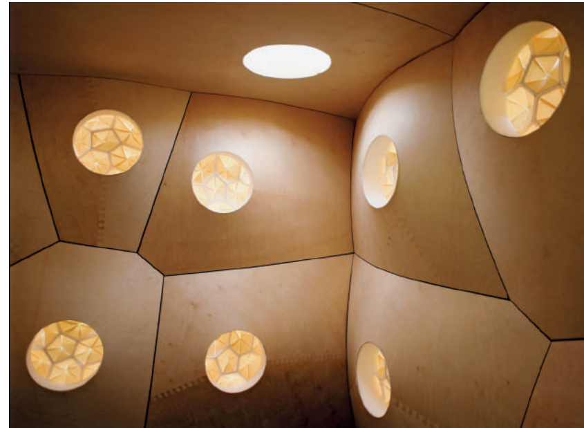
Fig. 5: Intersecting conical geometries. Interior view of the HygroSkin Pavilion.
