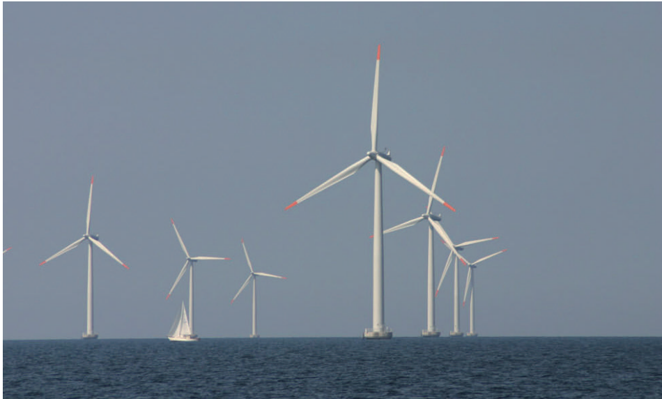
■ Photo 29 : the Horns Rev offshore wind farm on the eastern coast of Jutland (80 wind turbines; 160 MW) where impact studies were conducted for 6 years (© Dong Energy, DK).
