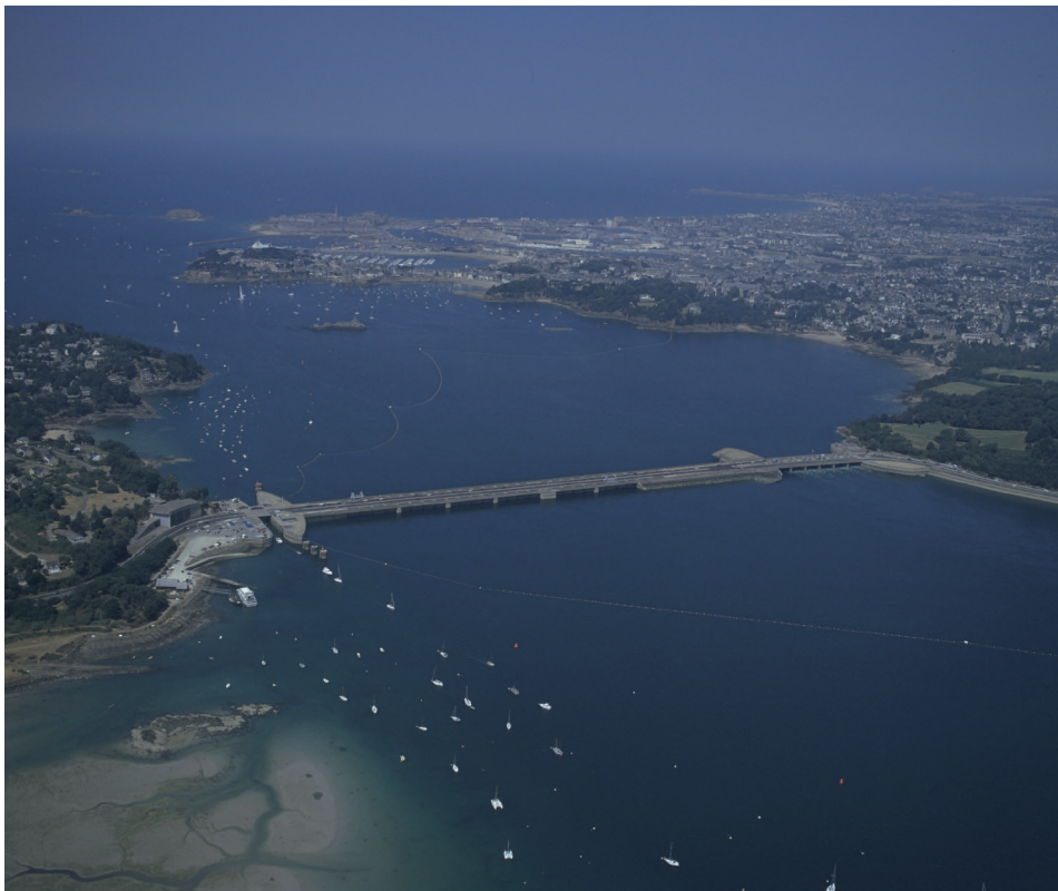
■ Photo 31 : aerial view of the Rance tidal power plant near St-Malo in Brittany (France) (© Médiathèque EDF).
