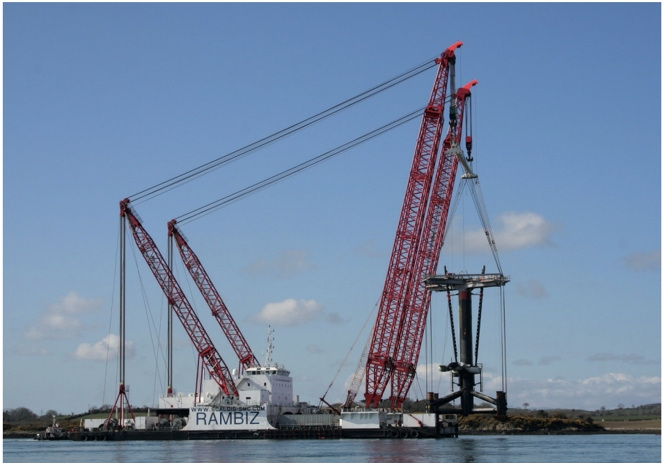
■ Photo 3 : Rambiz crane-barge installing the Seagen stream turbine on the Strangford Narrows site, Northern Ireland (© Marine Current Turbines, UK).
