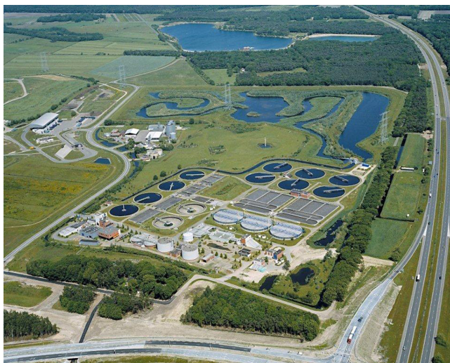
Figure 13.2 Overview of the STP Tilburg.
