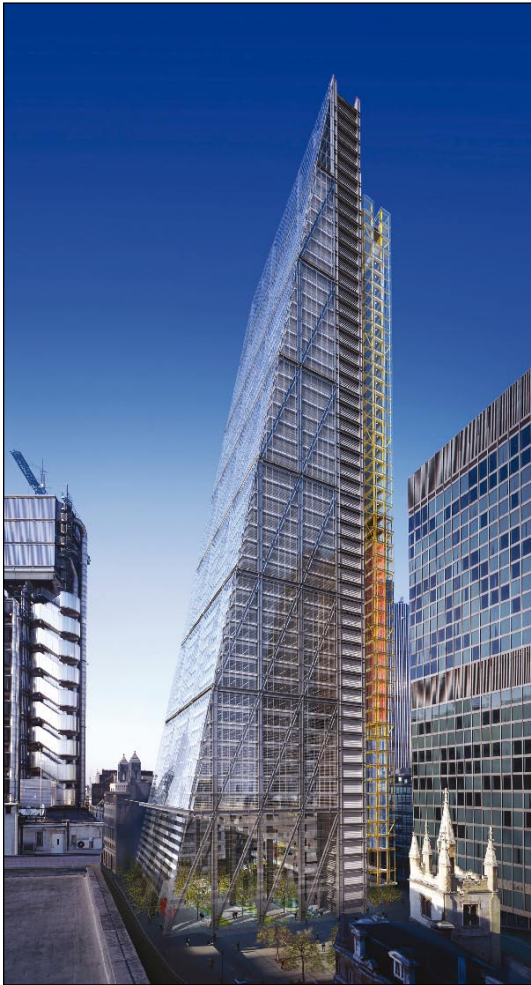
Fig. 15 Grattacielo a Leadenhall Street, Londra: vista della torre da Leadenhall Street (RRP - Cityscape).
