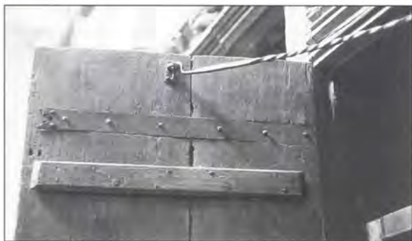
6.14 St Albans Cathedral, watching loft, detail.
