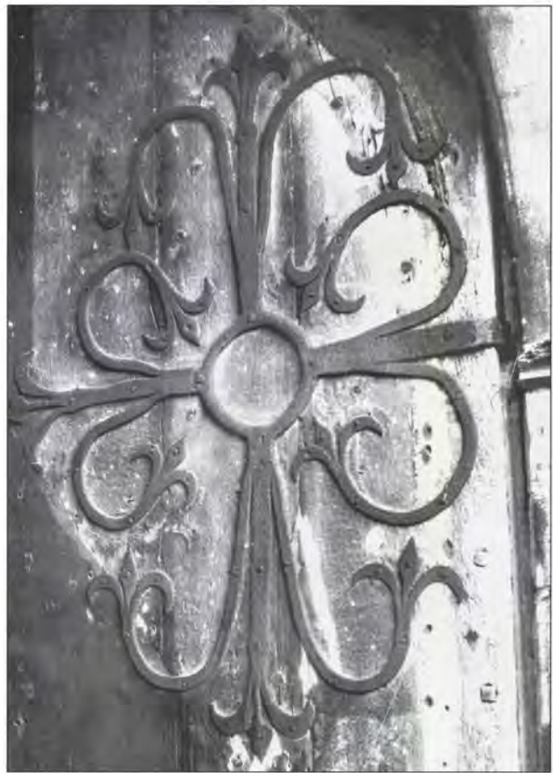
4.193 Beaulieu Abbey, refectory (now parish church), detail.
