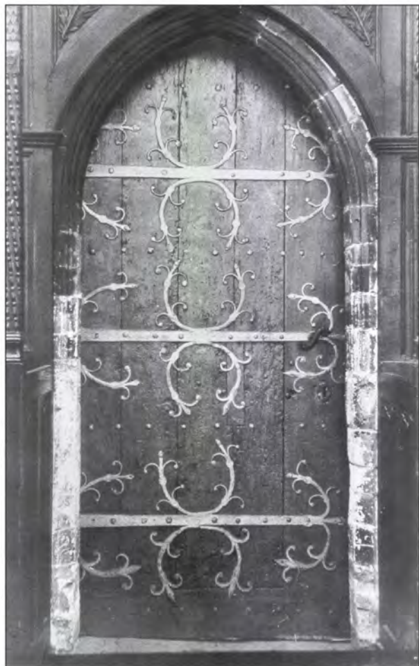
4.137 Winchester, south transept.
