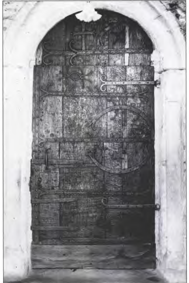
4.16 Old Woking, west, exterior (photograph: © Crown Copyright, RCHME).
