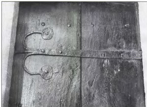
5.163 Low Ham, tower, interior (detail).
