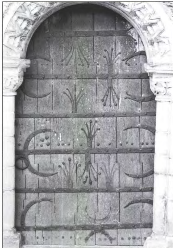
4.128 Edstaston, nave, north.
