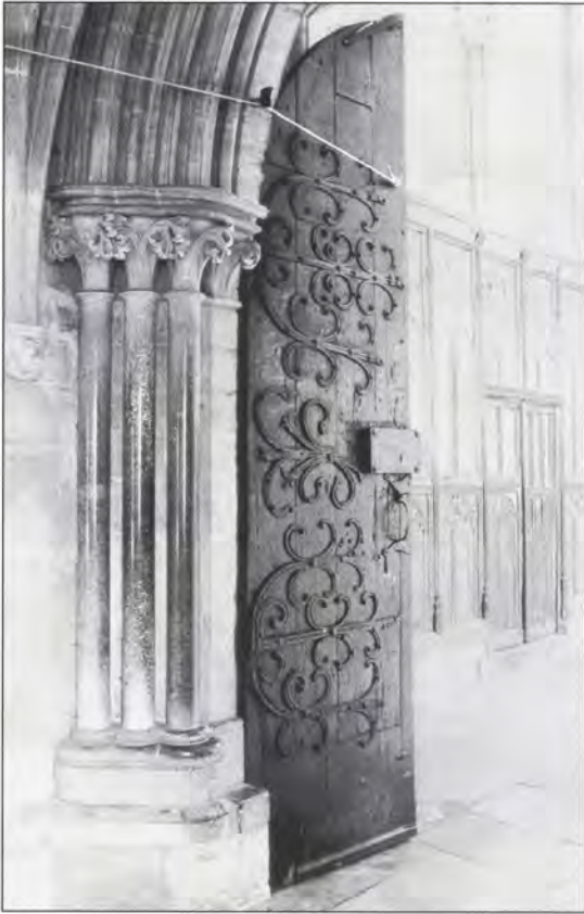
4.145 Lincoln, north-east transept, north wall (doorway from cloister).
