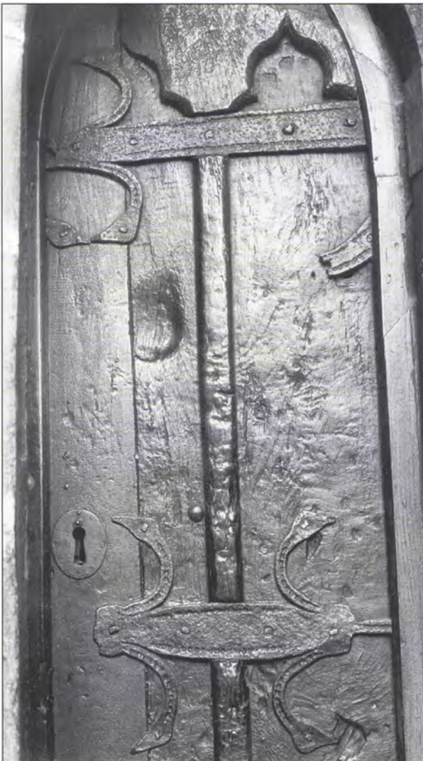
5.158 Ashbourne, south transept, doorway to rood loft.
