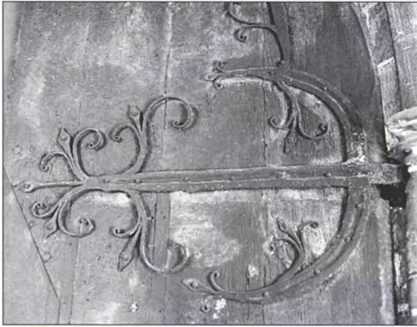
4.131 Thornton Curtis, south, detail.
