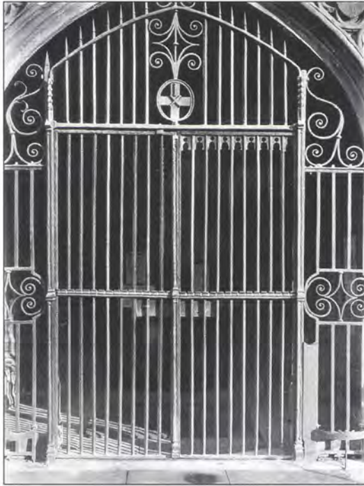
6.124 Canterbury Cathedral, grille from the nave, now in south-west porch (photograph: © Crown Copyright, RCHME).
