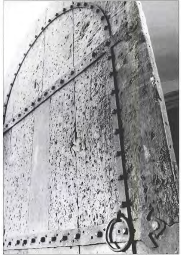
4.7 Hadstock, north, detail. Original exterior surface of wood and repaired ironwork.
