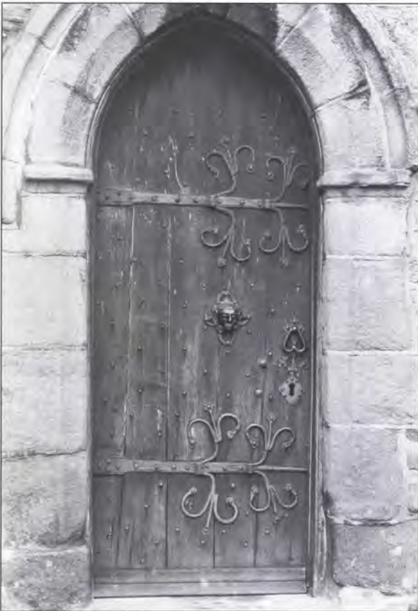
5.75 Whalley, St Mary, chancel south (photograph: B T Batsford Ltd).
