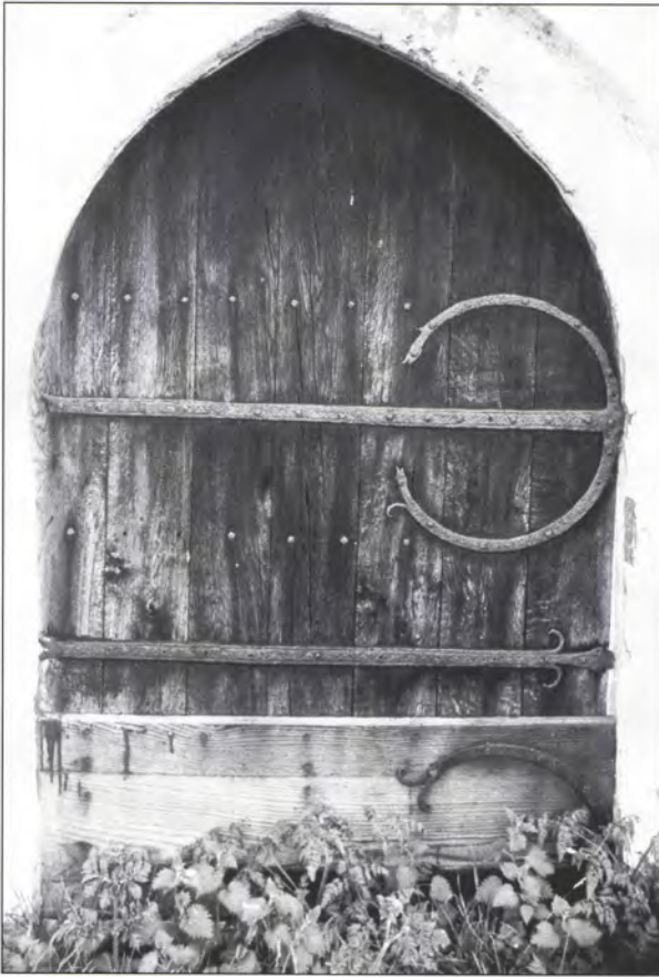
4.54 High Roding, north.
