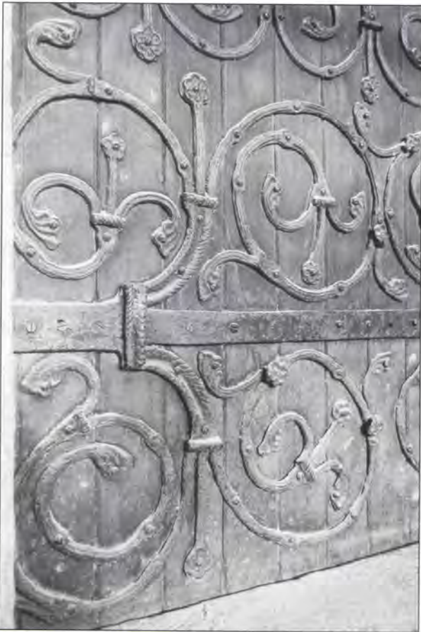
5.37 Eaton Bray, south, showing detail of welds.
