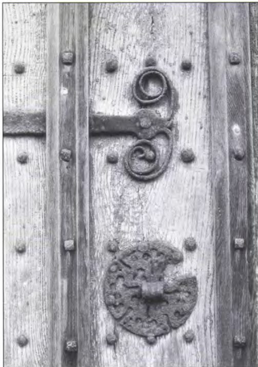
4.160 Burford, Oxfordshire, south aisle, west (detail).
