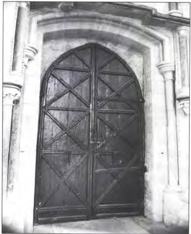
2.6 Lincoln Cathedral, north-east transept, north wall, doorway to cloister, rear frame.
