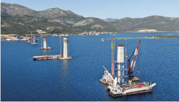
Fig. 4.10 Construction site of the bridge
