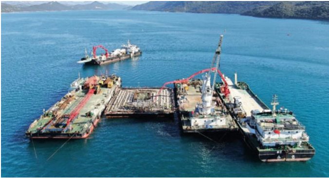
Fig. 4.15 Main construction materials and equipment meet CE certification
