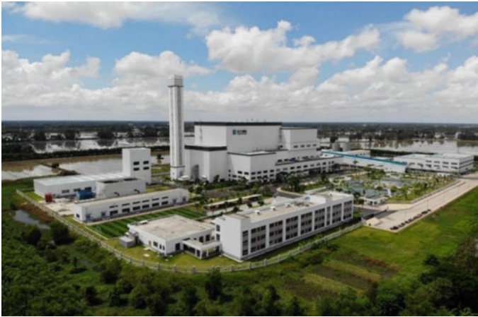
Fig. 5.1 Panorama of Can Tho waste-to-energy plant in Vietnam
