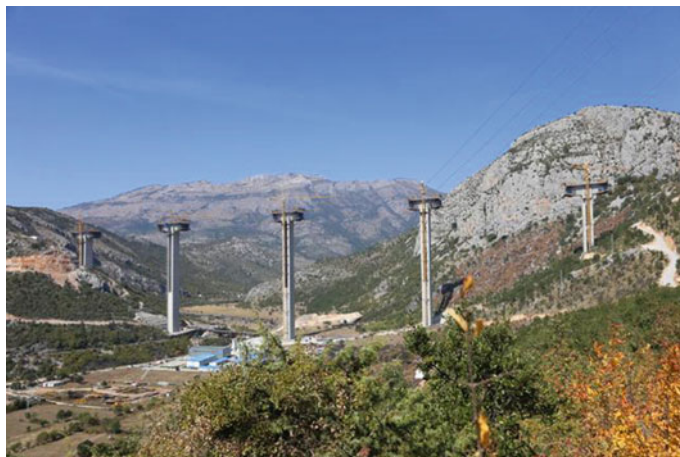
Fig. 4.2 Construction site of the Podgorica bridge (2018)
