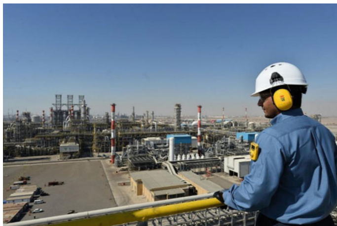
Fig. 6.4 A panoramic view of the Yanbu Refinery
