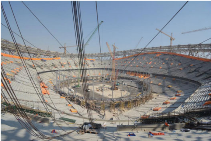
Fig. 7.2 The construction of the cable net roof
