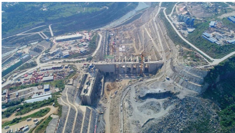
Fig. 2.2 Construction of the spillway
