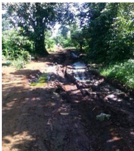
(a) Before the Repair
