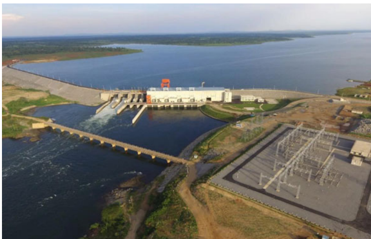
Fig. 9.2 Aerial view of the Isimba hydropower plant
