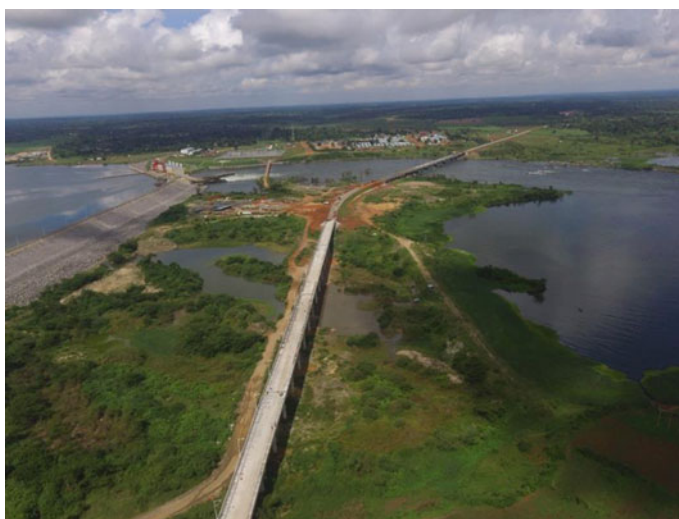
Fig. 9.3 The downstream public bridge
