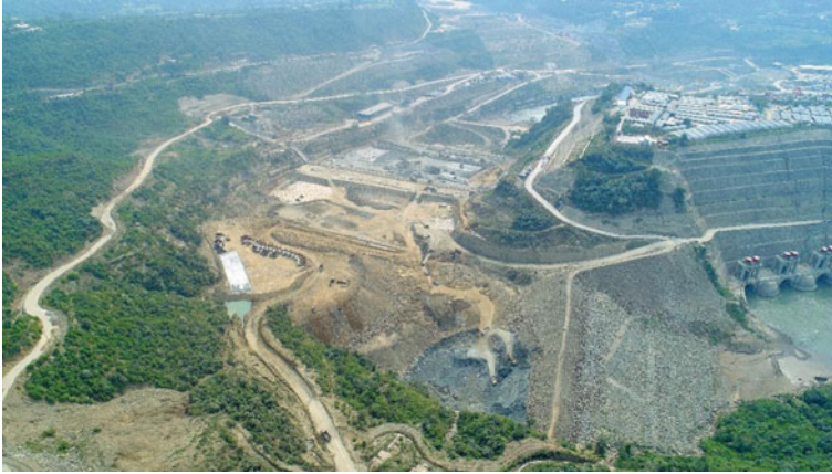
Fig. 2.3 Construction site of the dam zone
