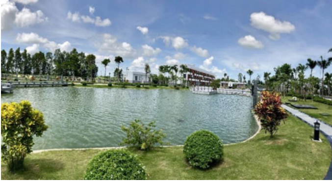
Fig. 5.3 The Can Tho waste-to-energy plant in Vietnam
