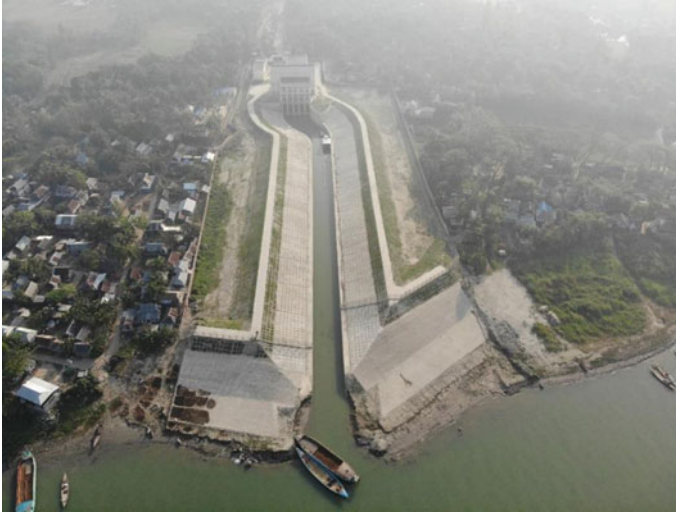
Fig. 3.13 Aerial view of intake facilities
