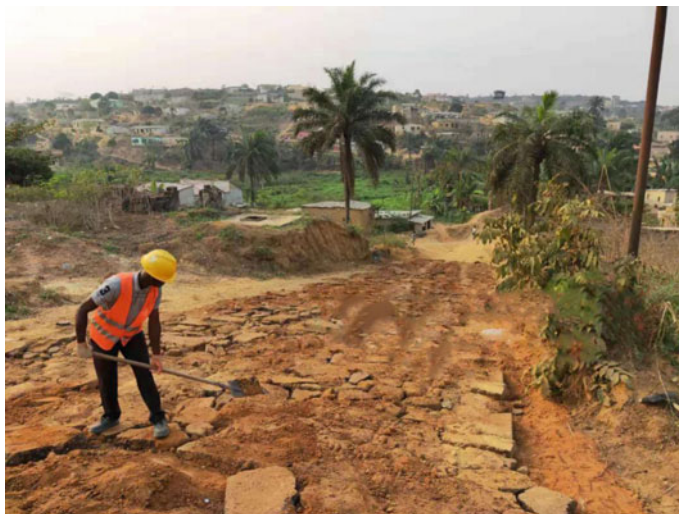
Fig. 3.4 Use of waste bituminous concrete to protect steep road segments from runoff
