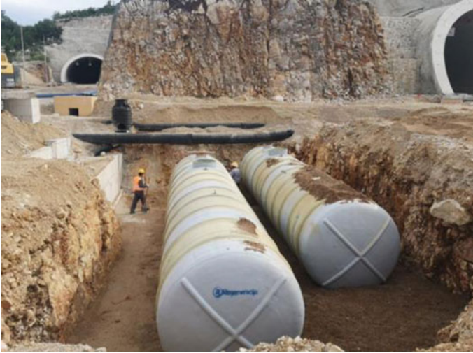
Fig. 4.7 Installation of oil–water separators
