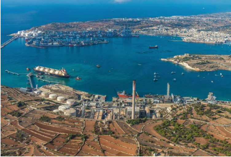
Fig. 2.8 D3 power plant in Malta
