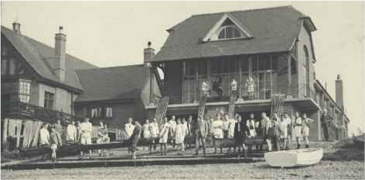
Fig. 87 The Polytechnic Boathouse was to suffer significant bomb damage during the Second World War and the boats were destroyed by fire.
