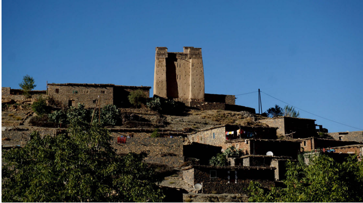
Figure 6: Restored ighrim of Amezray (upper village)
