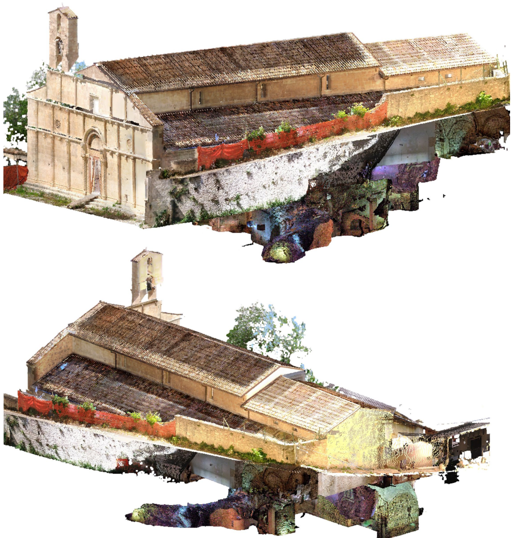
Fig. 3. Three-dimensional views of the point cloud.
