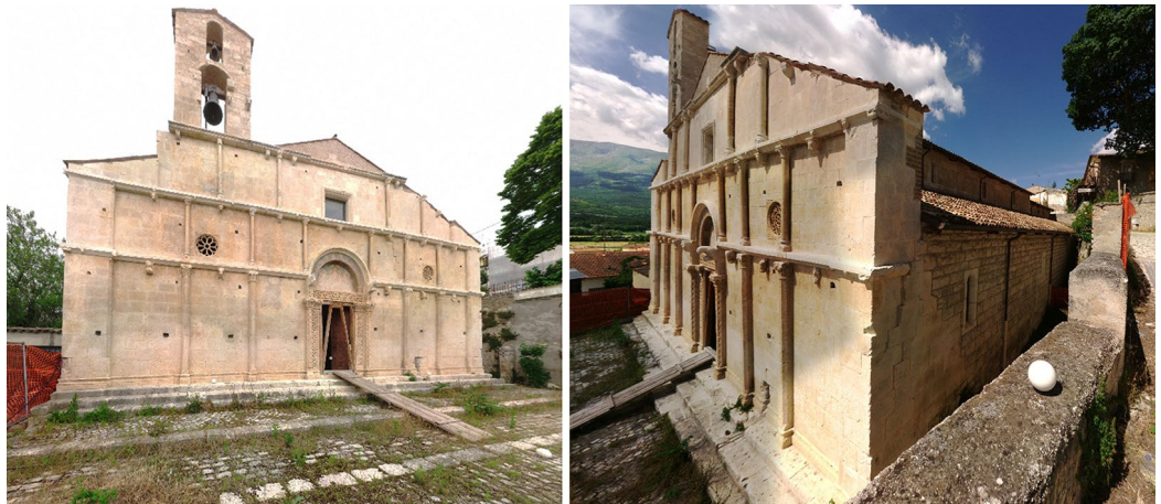
Fig. 1. The church of St. Giusta in Bazzano, near L'Aquila.
