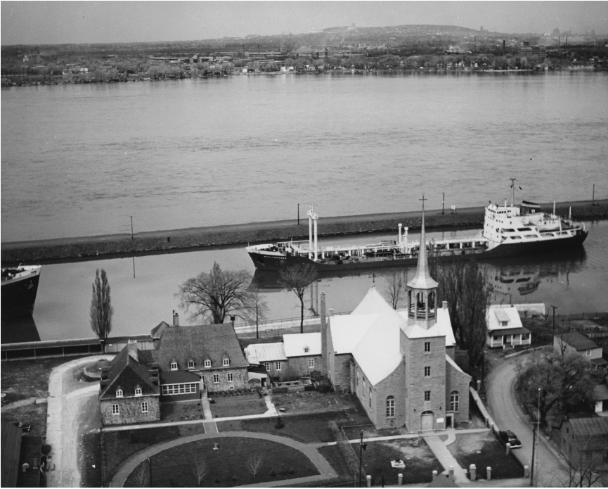
FIGURE 9.2. St. Lawrence Seaway lock across from Montreal. Used with permission of Library and Archives Canada.
