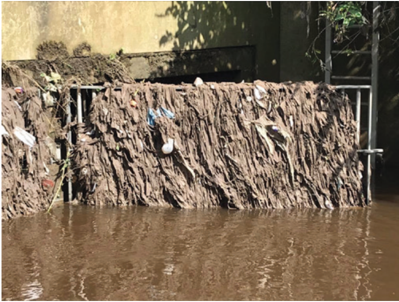
Figure 6.4: Penny Lane Grimesbottom combined sewer overflow, flowing into River Tame, Stockport, Greater Manchester
