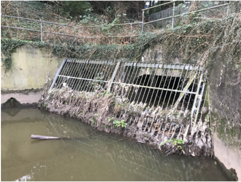
Figure 6.3: Liverpool Road/Newhall Avenue combined sewer overflow, flowing into Salteye Brook, Eccles, Salford, Greater Manchester
