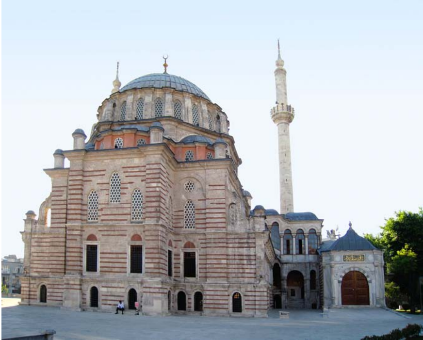
FIGURE 11.10 Laleli Mosque, Istanbul, 1174–1177/1760–1764, qibla façade of the prayer hall, with the royal pavilion on the right AUTHOR'S PHOTO
