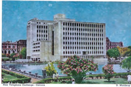
Fig. 34: Kolkata, New Telephone Exchange.
