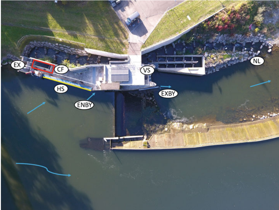
Fig. 5.1 HPP Schiffmühle, River Limmat. VS: vertical-slot pass, NL: nature-like pass, EX: exit of fishpass, CF: counting facility of the fishpass, HS: horizontal bar rack, ENBY: entrance bypass, EXBY: exit bypass
