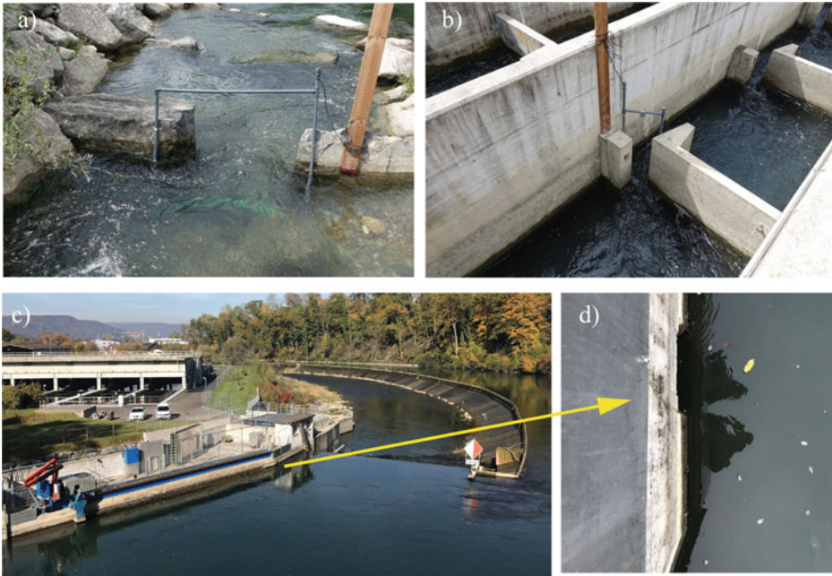
Fig. 5.2 a PIT-tagging antenna in the nature-like fishpass, b antenna in the vertical-slot pass, c turbine inlet with horizontal bar rack and d close-up photo of bypass system
