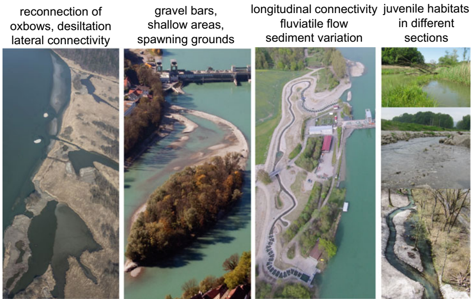
Fig. 14.2 All habitat components need to be available and reachable to meet the whole set of requirements of the life cycle. Nature like bypass channels can play a major role to add components to the anthropogenic changed river system
