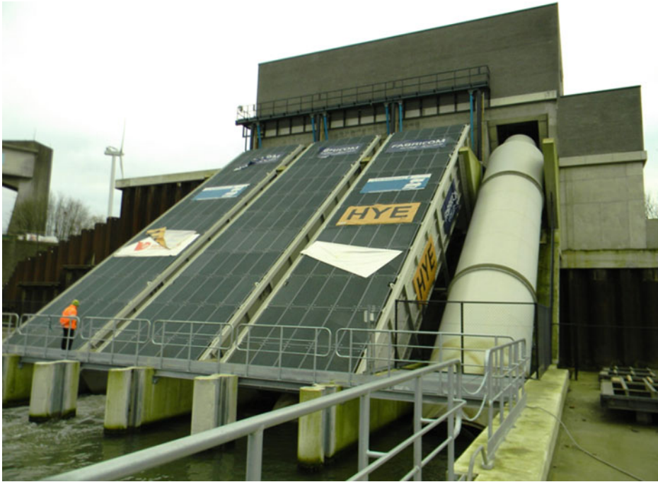
Fig. 11.1 The hydropower station of Ham (Belgium), equipped with three Archimedes hydrodynamic screws (on the left; the cover does not turn with the screw and is fixed; the screws can pump water and generate power as turbine), and one true Archimedean screw (on the right, the cover is fixed to the screw and turns with it; this screw can only pump water)
