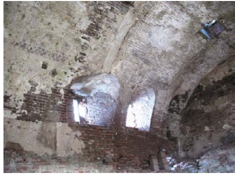
Figure 2 – The barrel-vaulted room with remains of plaster with red decorations (older part of the fortress).
