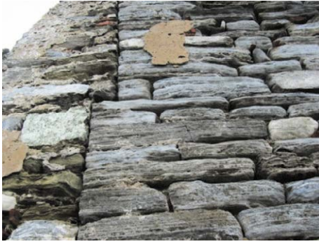
Figure 4 – The buttress and the corners in calcschists.
