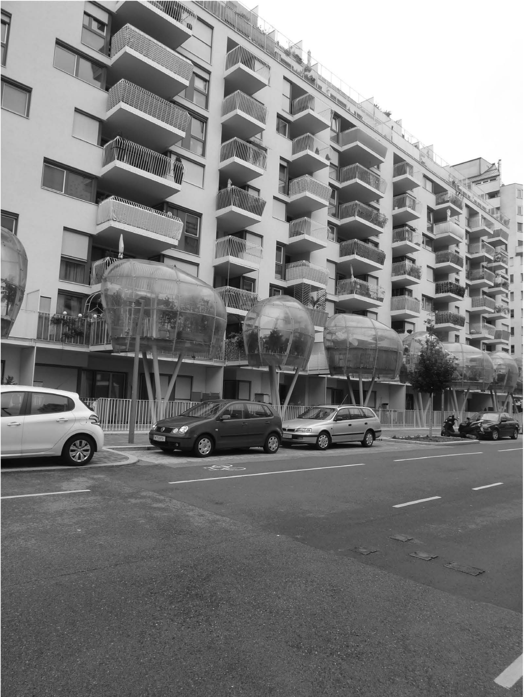
FIGURE 3.7.3 Bike and Swim development in the Nordbahnhof area, Vienna (master plan 1992, building designed in 2012 by Günter Lautner/Nicolaj Kirisits). This municipally financed social housing project offers communal bike sheds, a sauna, a fitness room, a sun deck, and a spectacular pool on the roof with a view across the city. Rents are affordable, set at approximately 550 euros per month for an 80-square-meter two-room flat in 2012 (author).
