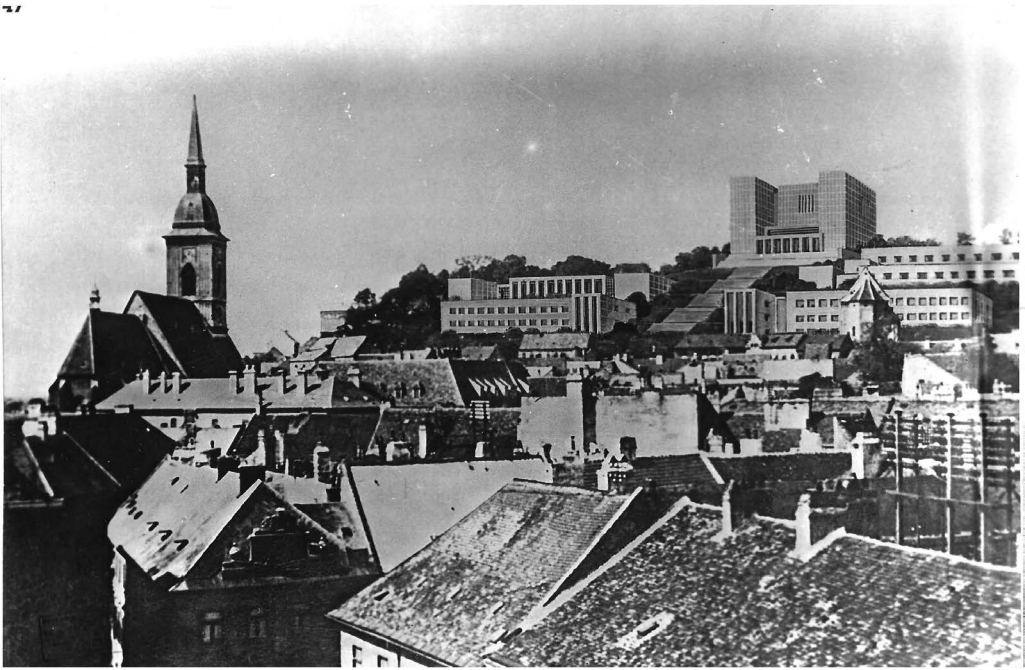
FIGURE 2.2.1 Ernesto La Padula, Attilio La Padula: Competition proposal for the University City in Bratislava 1940–1941 – 2nd prize ex aequo.
