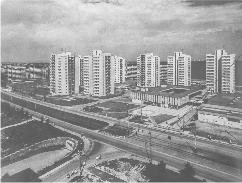
FIGURE 2.6.5 Rapid tram in the new residential area Výškovice in Ostrava, planned in the 1970s. The tram line was located in the center of an urban road (Výškovická) where prevailed road traffic conditions and which impeded pedestrian access to tramway stops.
