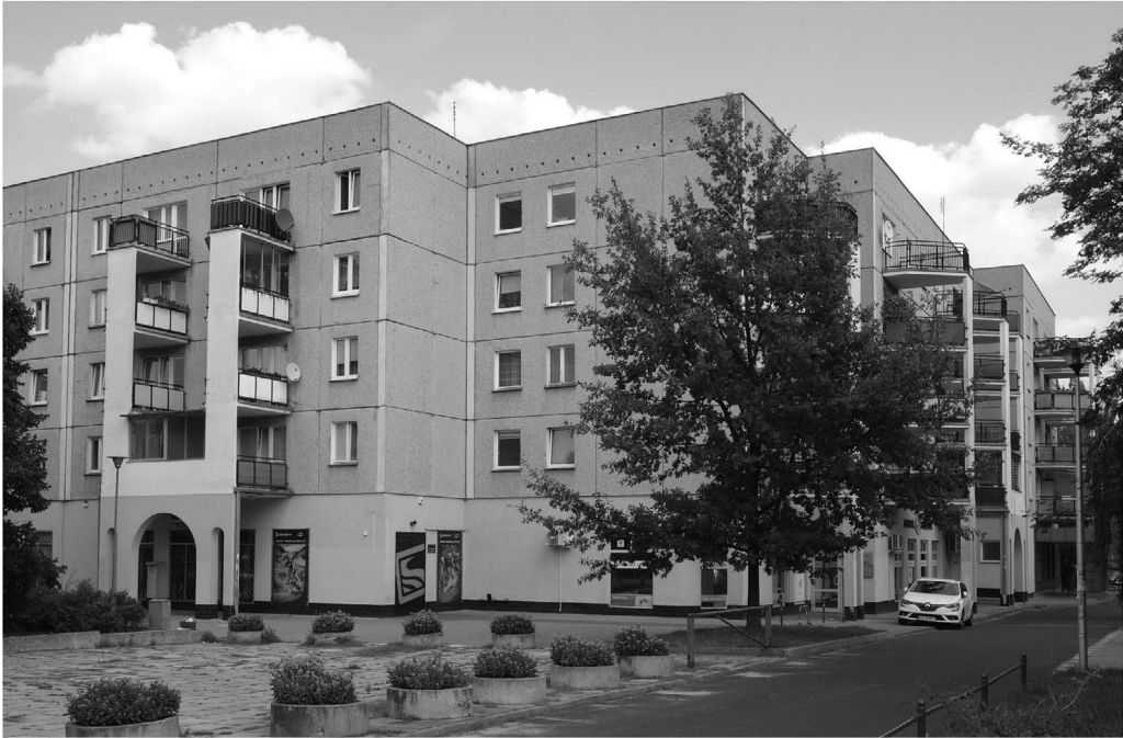
FIGURE 3.7.1 Socialist mass housing from prefabricated panels in Warsaw-Ursynów, Zamiany Street (master plan 1971, building 1988–91 by Krzysztof Kasperski), owned by the housing cooperative Spółdzielnia Budownictwa Mieszkaniowego Ursynów (author).
