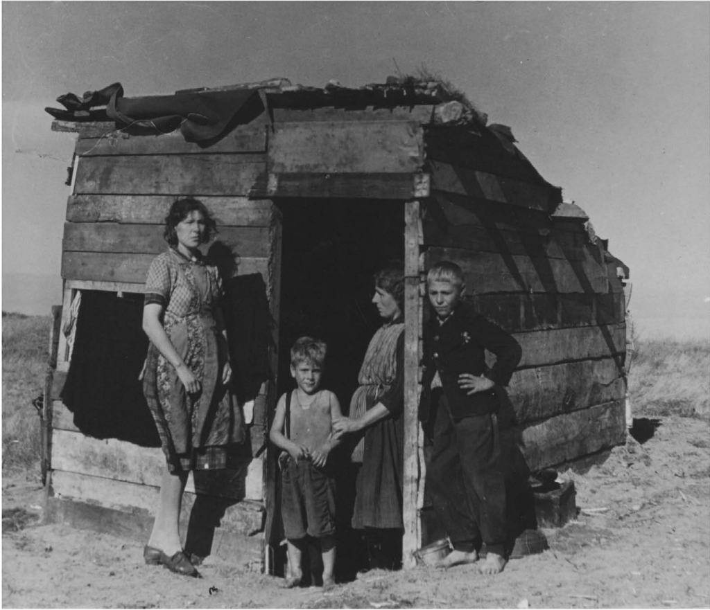
FIGURE 1.3.4 Shacks in Limburg, the Netherlands, known as “krotten”, 1945.
