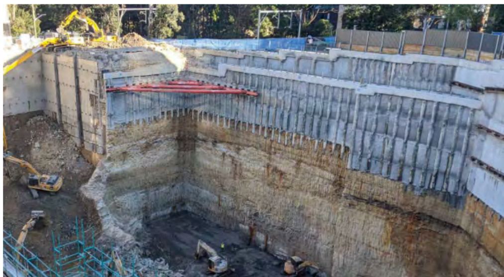
Figure 5. Excavation support along Sydney Trains (west) boundary.
