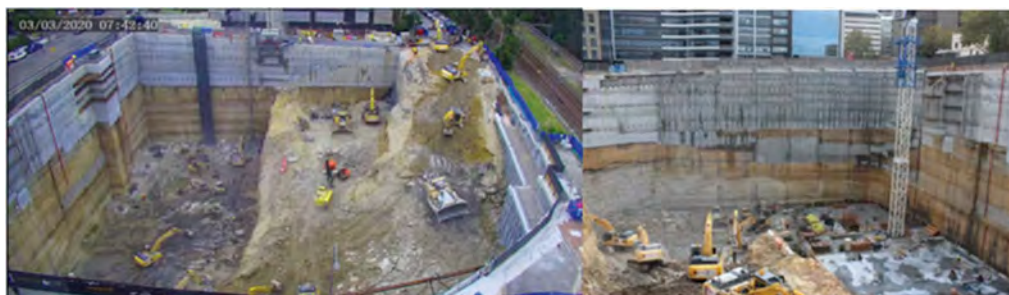
Figure 9. Bulk excavation works - view to south and north.
