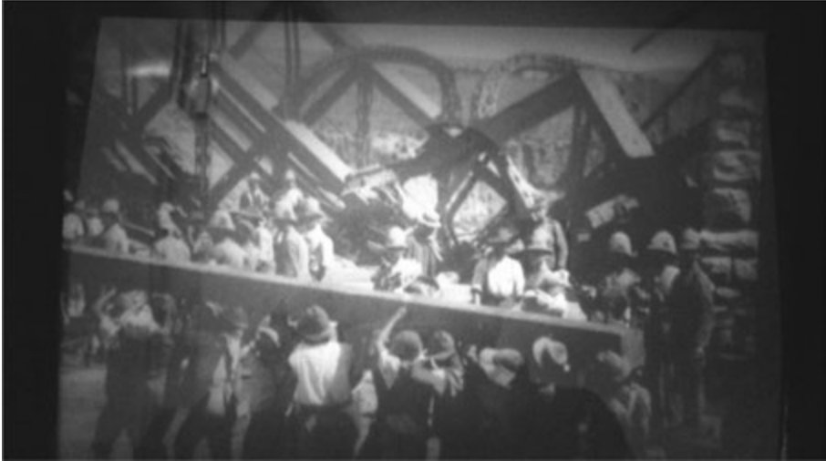
Figure 5.9. Still from Repairing the Broken Bridge at Frere , 1899, shot by WKL Dickson, British Mutoscope and Biograph. Source: South African National Film Archive, Pretoria.
