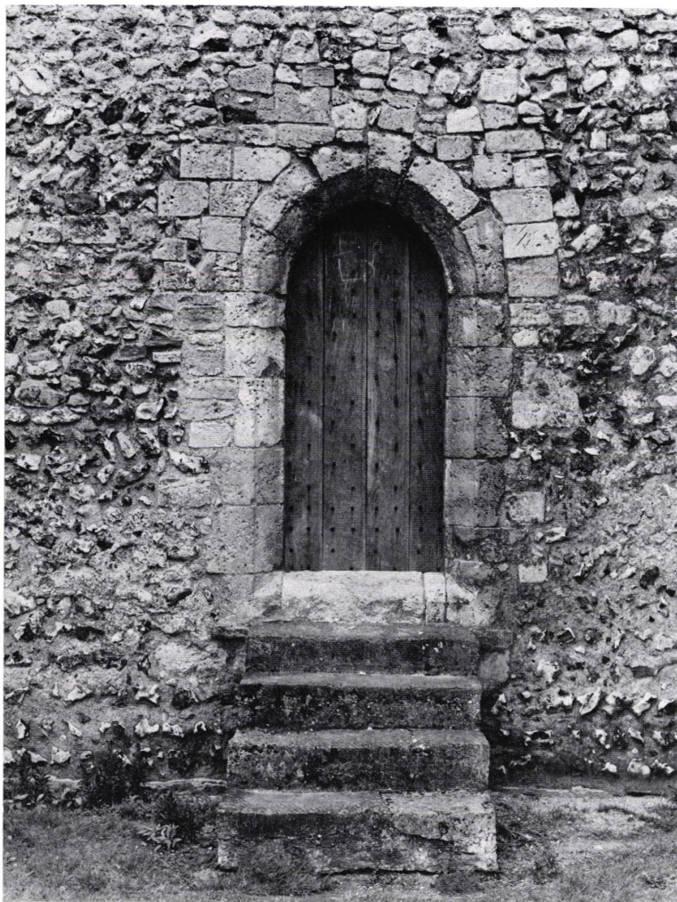
a. The north postern from outside the fort (pp. 93, 97)
