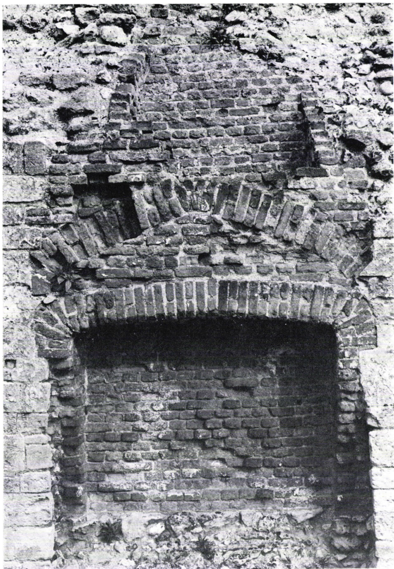
a. Fireplace in first floor of east range: seventeenth century (pp. 51, 119)
