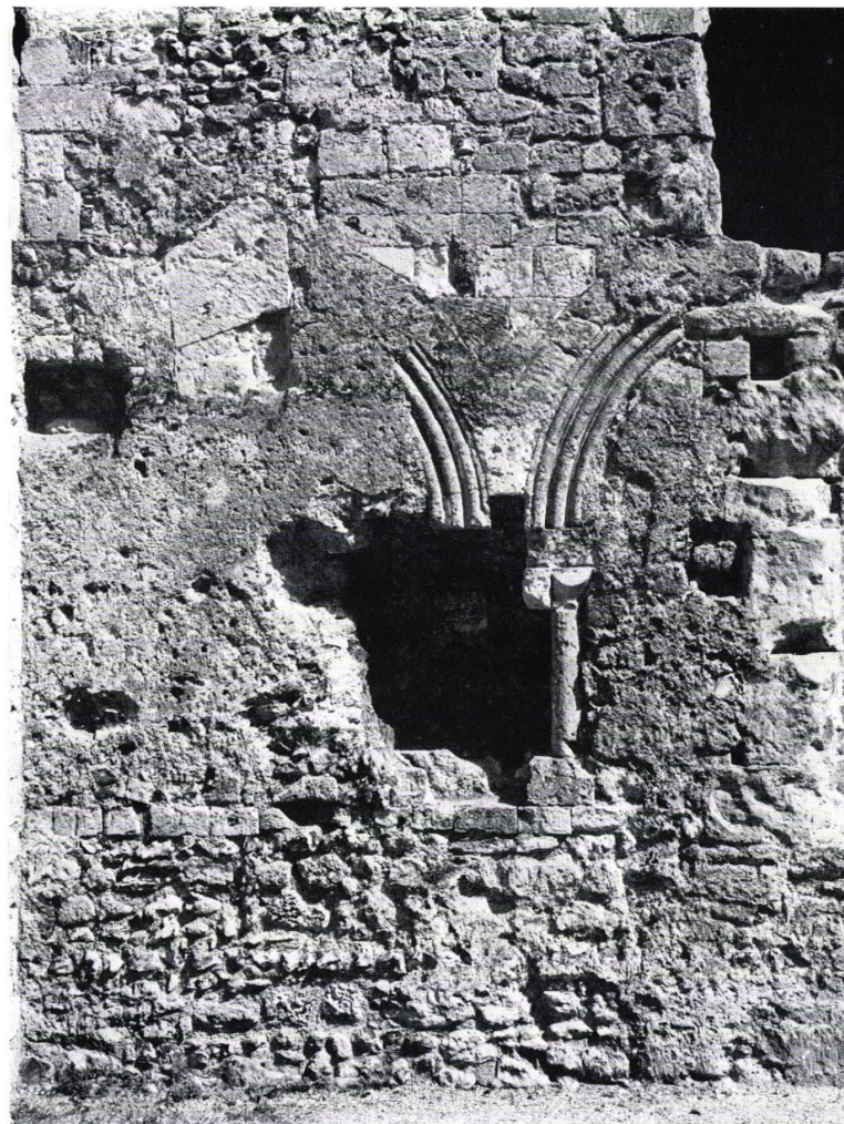
b. Norman windows or arcade in hall (south-west range) (pp. 17, 98-9)
