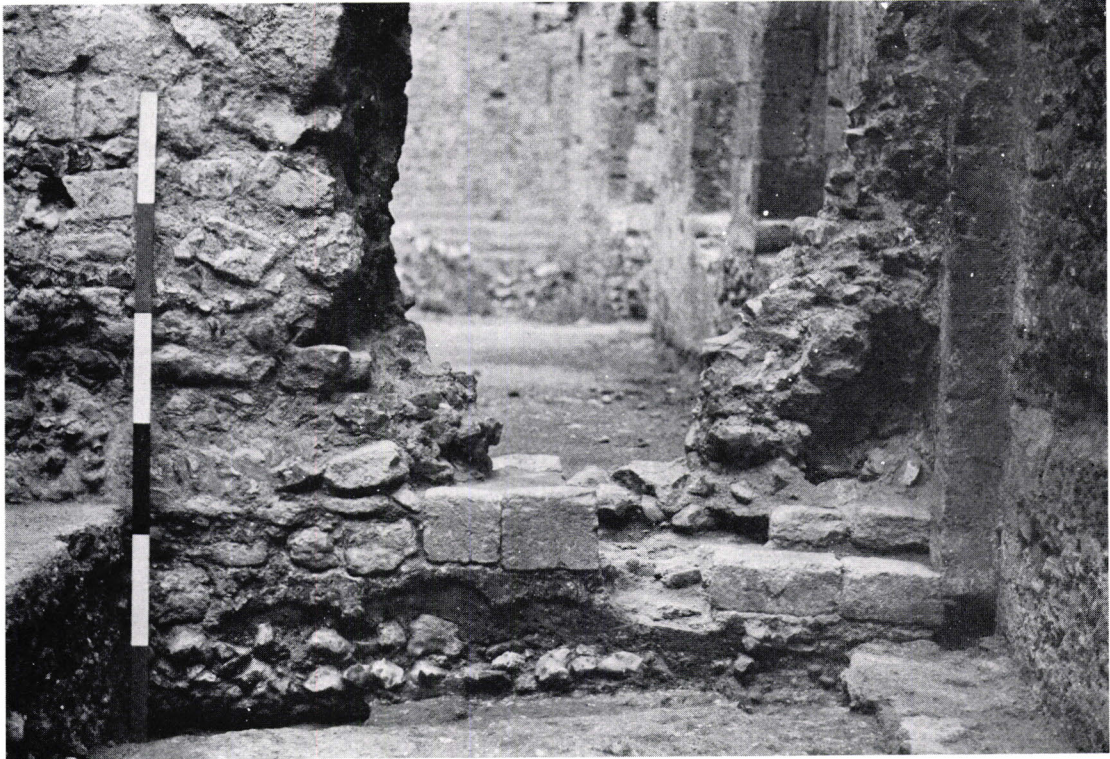
a. Footings of Norman door leading from the south-west to the west range in trench C36 (p. 17)
