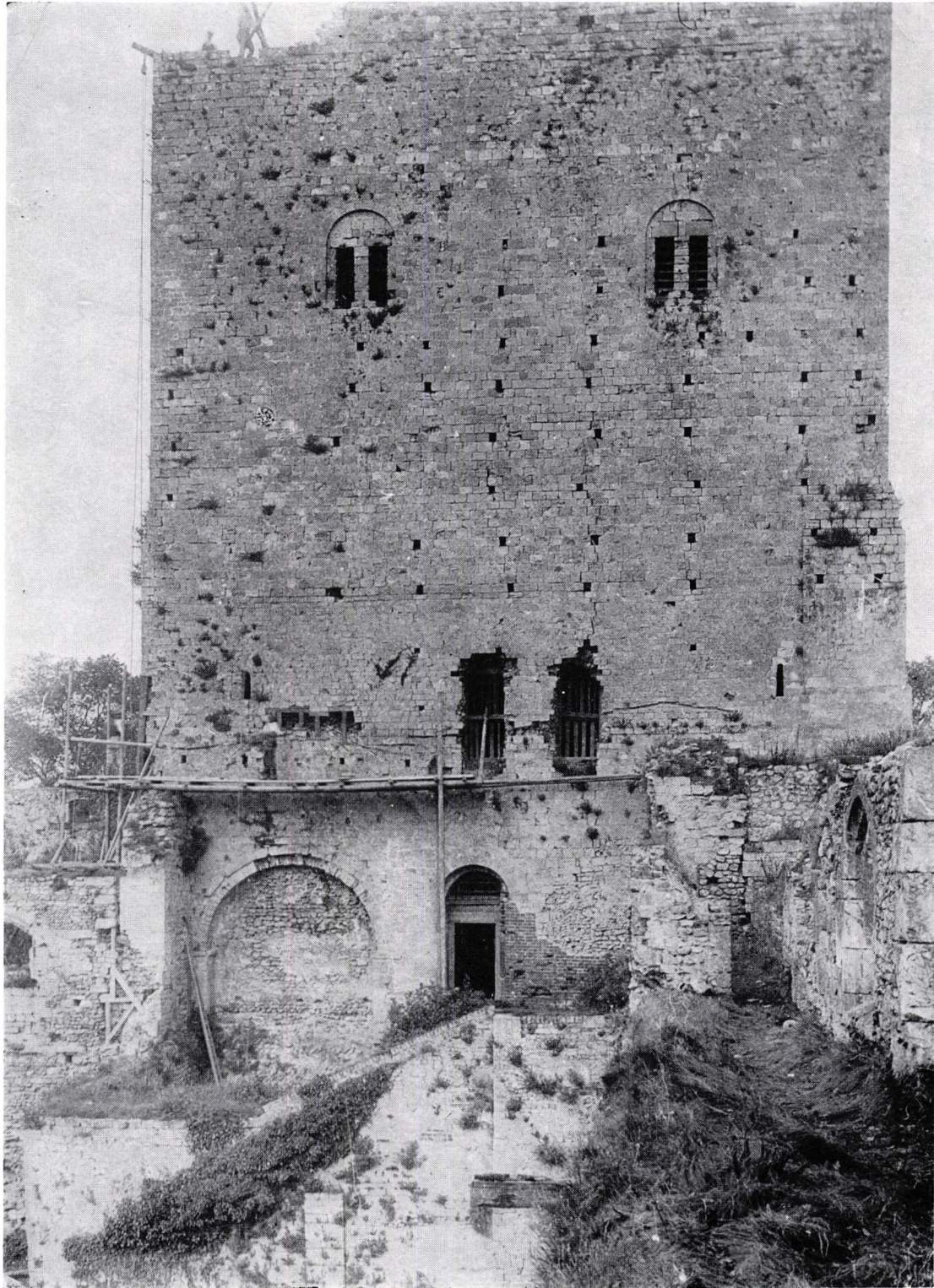
Keep: east face during restorations of September 1926. Note support wall for external staircase (pp. 12, 77, 78, 81, 82)
