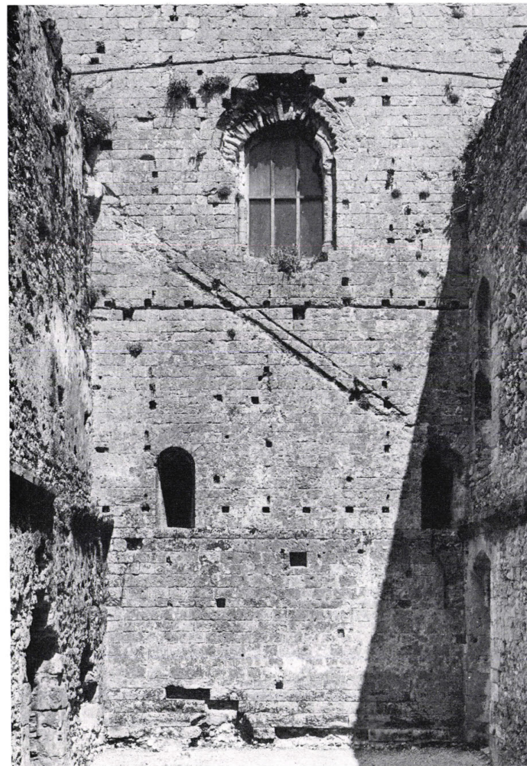
b. Keep: detail of south face showing roof lines of various dates (pp. 12, 78, 99)
