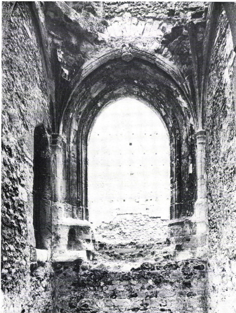
a. Door leading from the porch to the screens passage in the hall of south-west range (4) (p. 103) Photograph: Department of the Environment
