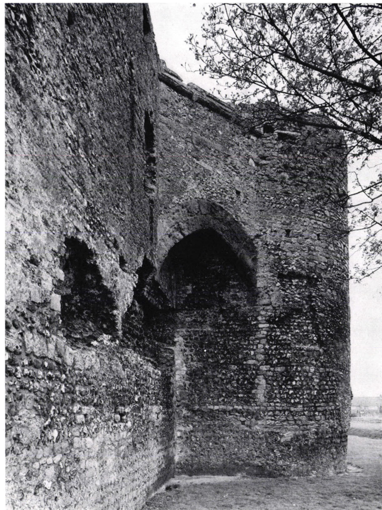
b. Squinch containing latrine shoots attached to the north bastion tower (pp. 95, 113, 115)
