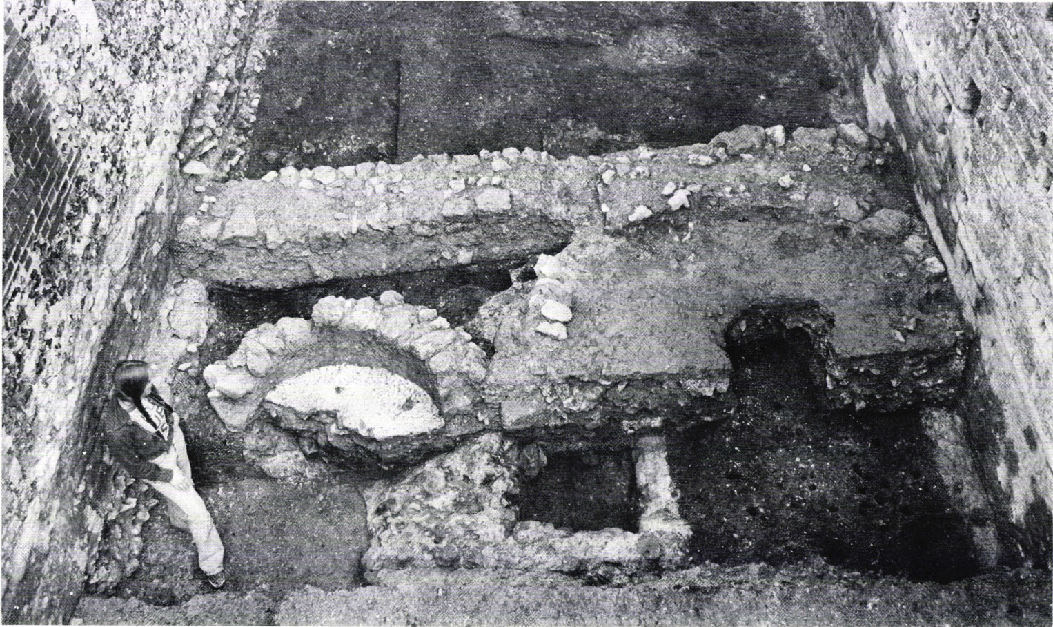
Oven and tank in east range in trench C45. Roman structure below (pp. 47, 69) Photograph: Mike Rouillard
