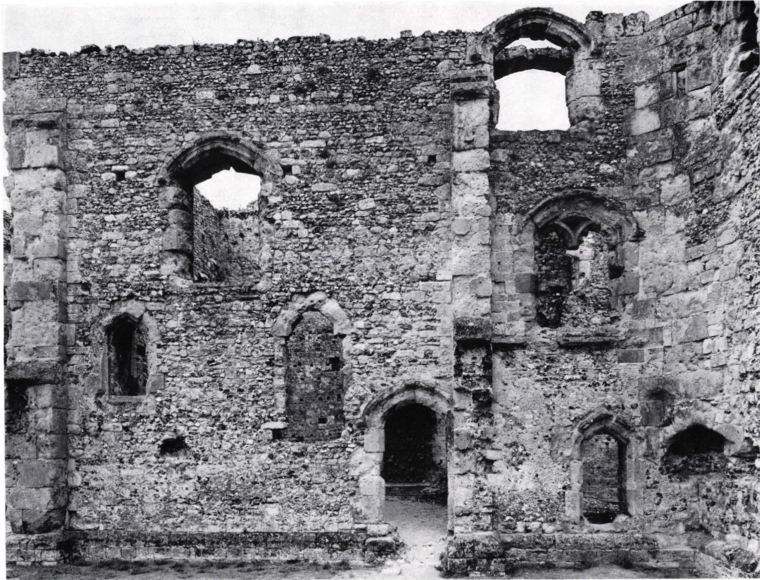
South-west range (4): north wall of kitchen (p. 101) Photograph: Department of the Environment
