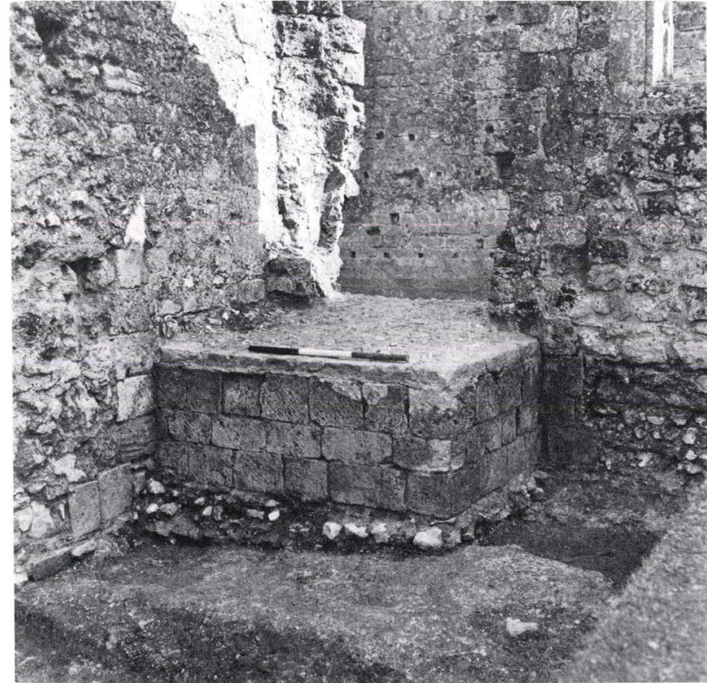
b. Chimney-breast for fireplace in south-east range in trench C50. The capping beneath the rod is modern (pp. 34, 49)
