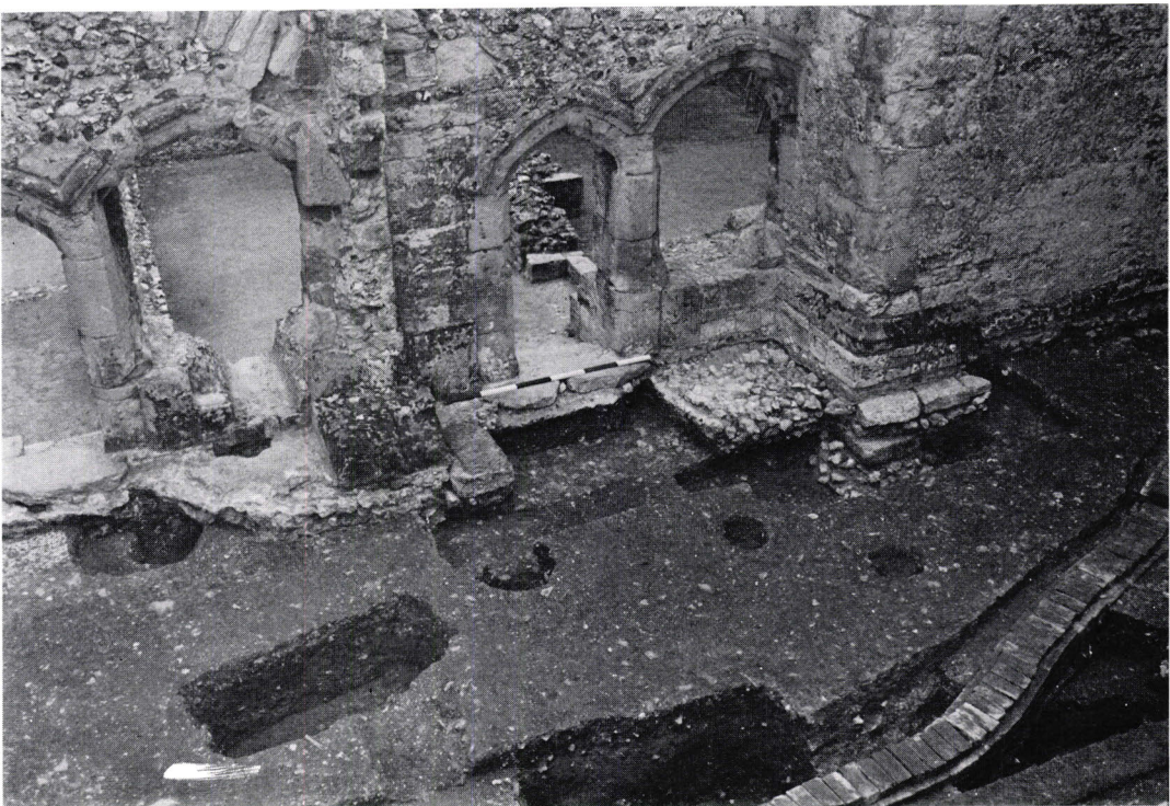
b. Footings of the south-west range exposed in trench C35 (pp. 18, 25, 30)
