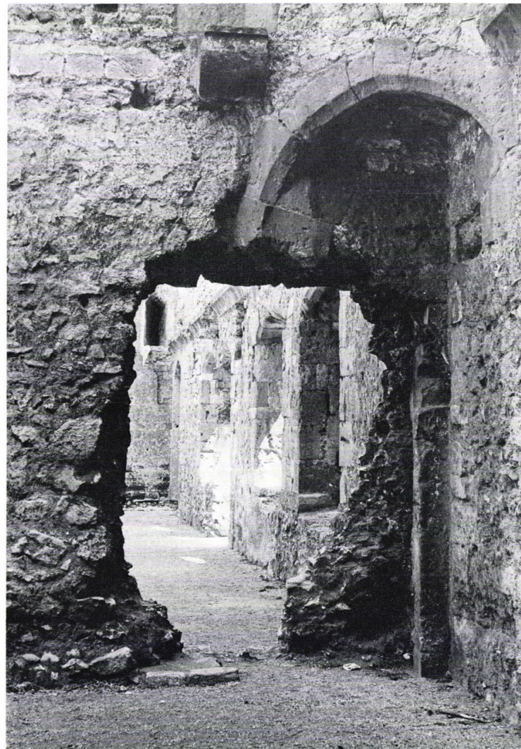
b. Chamber in the south-west corner of the inner bailey showing Norman door with some fourteenth-century blocking in position to support the squinch taking the spiral stair from the first floor passage to the roof (pp. 17, 100-1) Photograph: David Baker
