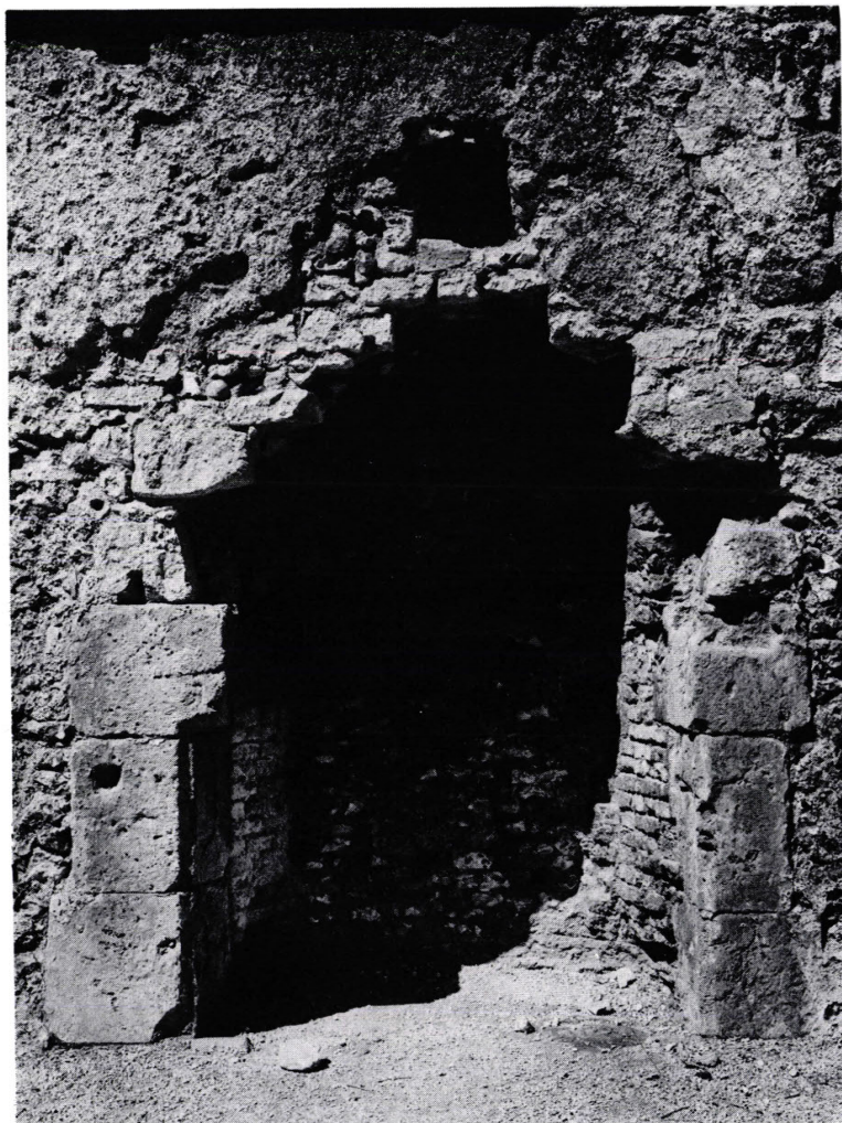
a. Late fourteenth-century fireplace in the north part of the west range (4), showing use of Flemish bricks (p. 108)
