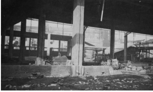
Figure 3. Sant'Elia Kindergarten, worksite with the structures in reinforced concrete completed (AT, 43/004/C/S ca.1936).
