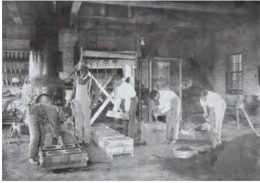
Figure 1. Tuskegee students learn to mix and pour concrete. Published in L. Albert Scipio II, The building of Tuskegee Institute (Silver Spring, MD. Roman Publications 1987): 241.
