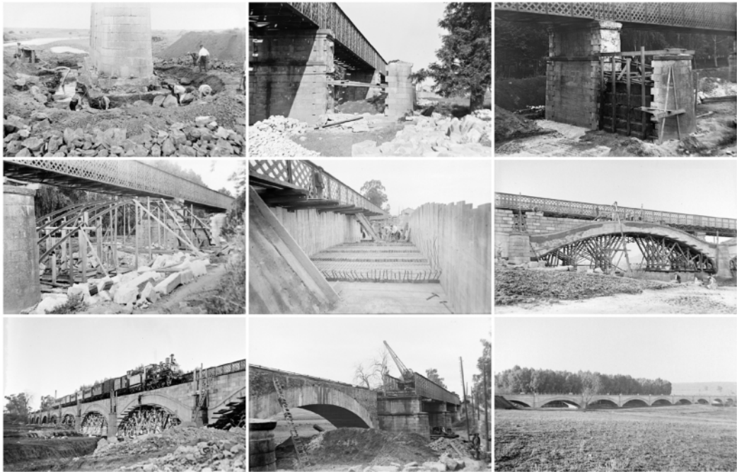
Figure 3. Aljucén Bridge. Top: soil excavation near the abutments; dismantled pier; rebuilt pier. Middle: centering; frame in the top of the arch; spandrel made of ashlars. Bottom: a train in the first half of the bridge; crane dismantling the metal bridge; new bridge already completed. Photos by Juan Salgado Lancha (AHF-MFM MZA- 0232-IF_10-20-; MZA-0276-IF_10-23-; MZA-0282-IF_10-23-; MZA- 0284-IF_10-23-; MZA- 0271-IF_10-22-; MZA- 0235-IF_10-20-; MZA- 0241-IF_10-20-, MZA-0250-IF_10-21-; MZA- 0229-IF_10-19-). The collection consists of 64 photographs taken from 29.09.1926 to 05.11.1929.
