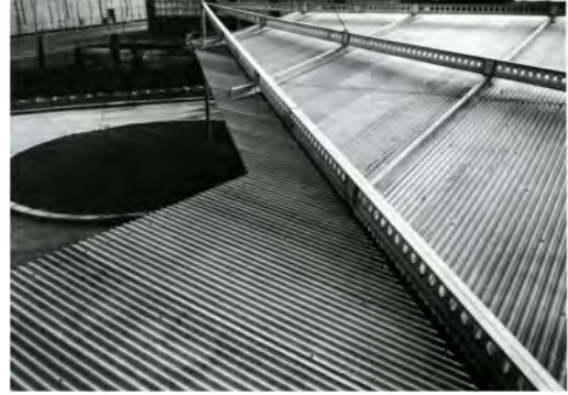
Figure 6. SEAT Dining Hall. Roof over the entrance hall comprising corrugated aluminium supported by aluminium I-beams. Archivo Histórico ETSAUN.
