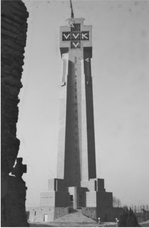
Figure 9. The new tower near completion during the placement of the lettering, ca. 1964 (Collection Karel Canfyn).
