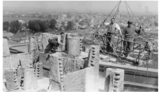
Figure 6. Prefabricated corner elements in place, ca. 1961 (Collection Karel Canfyn).
