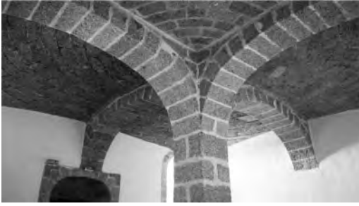
Figure 3. Vault in the basement of the Monastery of El Escorial.
