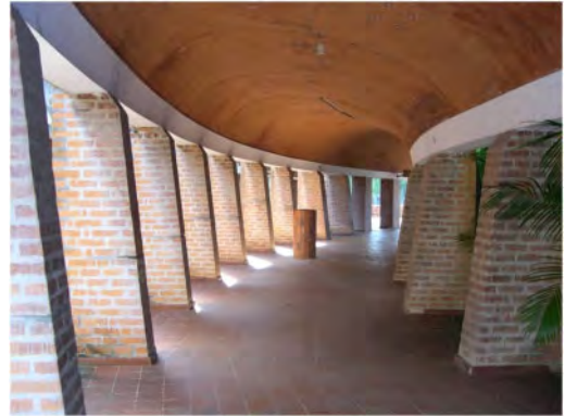
Figure 2. M. Paradiso (2006), detail of the buttresses supporting of the School of Plastic Art.
