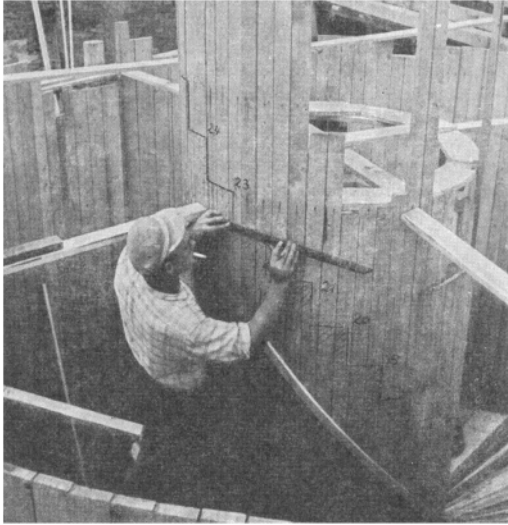
Figure 10. A formwork carpenter constructing a round staircase (Haerberlen & Kress 1959, 173).
