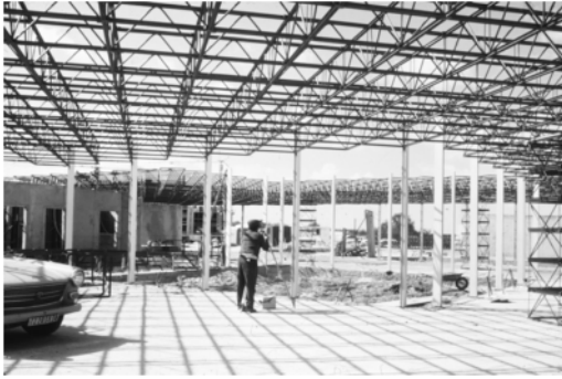
Figure 8. École Elancourt under construction.
