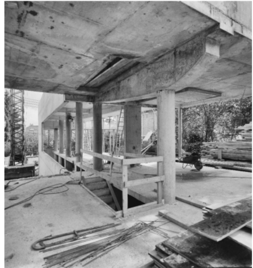
Figure 9. Cantilevered beam in construction (Hans Werleman).
