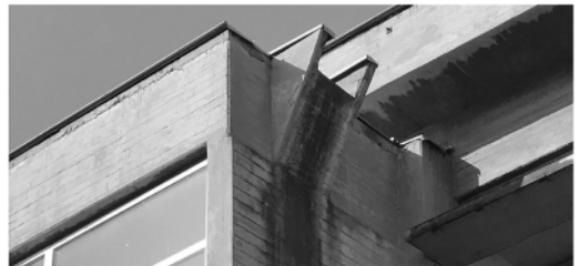
Figure 6. Flat-roof outfall in exposed concrete. Image: Iva Stoyanova, 2020.
