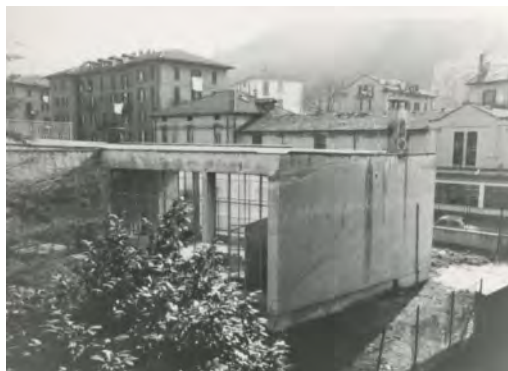
Figure 6. Diagonal cracks in the wall giving onto Via Alciato due to land subsidence (AT 25 February 1967).
