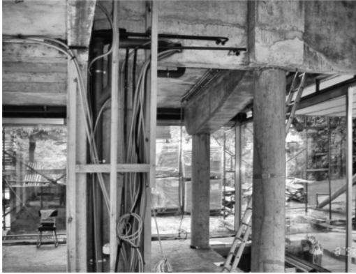
Figure 4. L-shaped pillar during construction (Hans Werleman).
