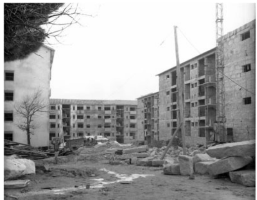
Figure 4. Outeiro . Rui Paixão, architect. Construction phase © Arquivo Municipal do Porto.
