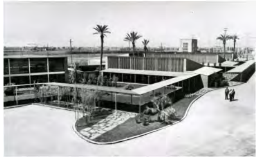
Figure 1. General view from the access. Archivo Histórico ETSAUN. (Historic Archive of the School of Architecture of the University of Navarre).
