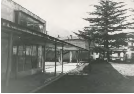
Figure 7. Provisional propping of the external cantilever roof (AT 25 February 1967).
