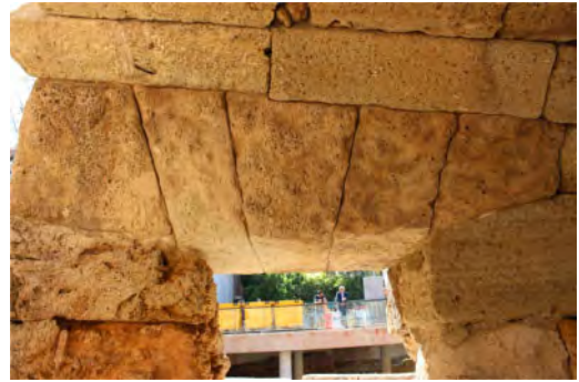
Figure 8. View of the lintelled arch (photo: R. García).
