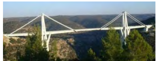
Figure 4. Wadi el Kuf Bridge, Libya (source: YouTube 2018).
