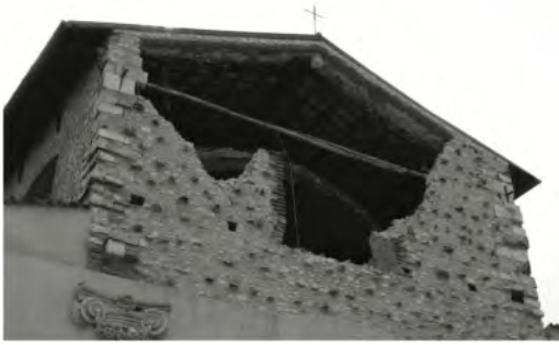
Figure 2. L'Aquila, chiesa di S. Giuseppe Artigiano, the metal anchors located in the corner walls connect the wooden 'radici-amenti'.
