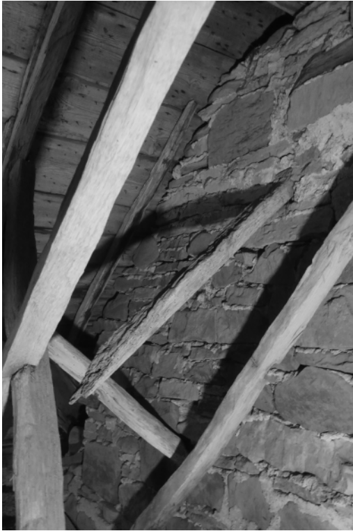
Figure 6. Remaining brace of a king post in the masonry gable crest of the chancel in Eriksberg church. Photo. R. Gullbrandsson.
