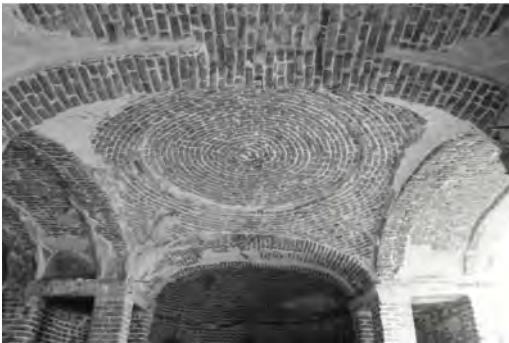
Figure 5. Northern vault in the Casa de Campo Garden Pavilion.
