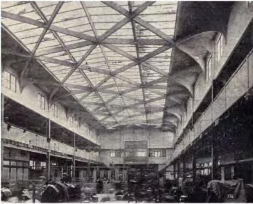
Figure 2. Factory roof, Paris. Design: Cottincin, 1900.
