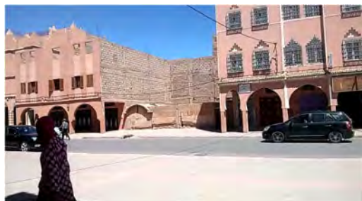
Figure 6. BTS 67 in 2018, Ouarzazate (photo: author).
