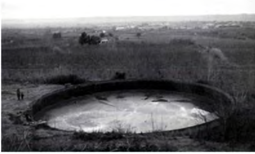
Figure 1. Open water tank in Puigverd, Lérida. Design: Francesc Macià. 1893.
