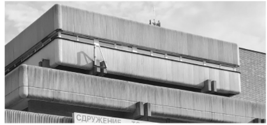
Figure 9. Almost identical parapet and façade panels. Image: Iva Stoyanova, 2020.
