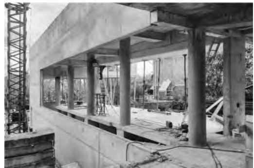
Figure 16. On site work. Façade north (Hans Werleman).
