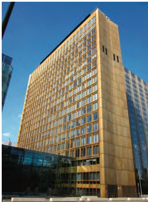
Figure 2. Curtain wall façade of the Axel Springer skyscraper (source: https://it.m.wikipedia.org/wiki/File:Berlin,_Kreuzberg,_Axel-Springer-Strasse_56,_Axel-Springer-Hochhaus_01.jpg ).
