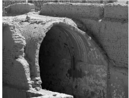
Figure 6. Barrel vault of the southern lateral nave (Lehmann).
