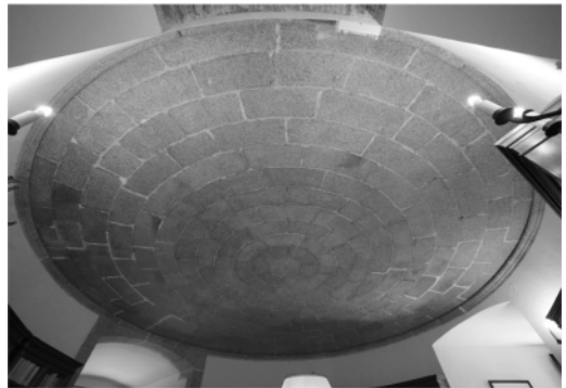
Figure 2. Vault in the ground floor of the Magalia Castle.
