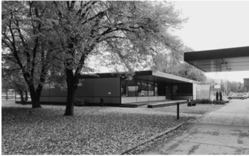
Figure 7. Current situation of the pavilion on the Gartner Campus. (Photo: A. Putz).
