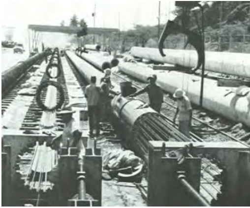
Figure 8. Track tensioned and manufacturing of the piles: already finished on the right; and placing the reinforcement and prestressing anchor on the left (source: Simons et al. 1963).
