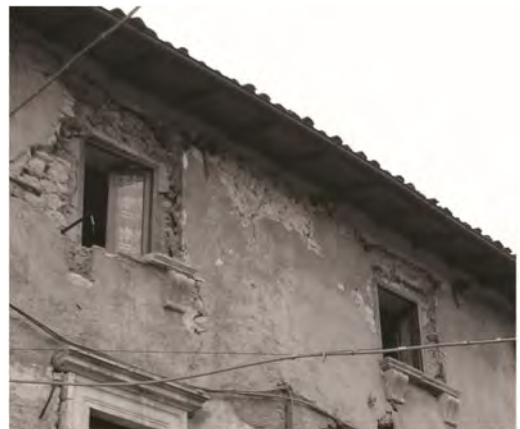
Figure 5. L'Aquila, wooden anchors of the roof trusses.
