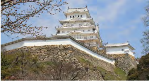
Figure 7. Donjon and stone walls of Himeji Castle. Source: author.
