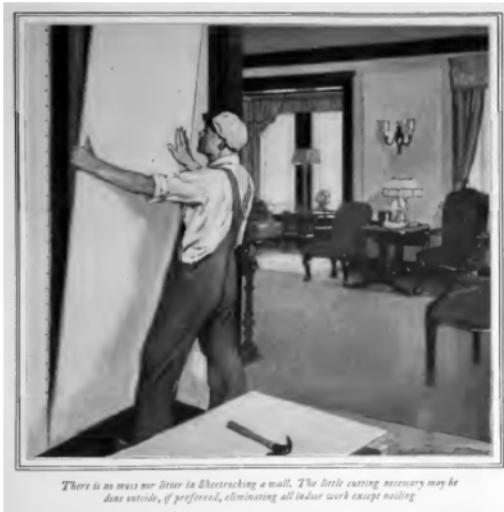
Figure 4. Sheetrock panel being installed by a single, semi-skilled worker. From USG, Walls of Worth (U.S. Gypsum ca. 1937).
