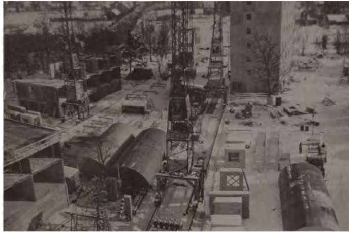
Figure 2. Construction site of Lassaskog buildings, Växjö. Air-heated Masonite hoods moved by cranes were used to cast concrete regardless of the weather. Construction continued through the Swedish winter. Photo: Sallstedts Bildbyrå / Nordiska museet.
