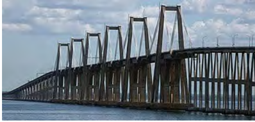
Figure 1. Bridge over Lake Maracaibo (1957–1962) (source: Taringa@ZuliaPrensa 2014).
