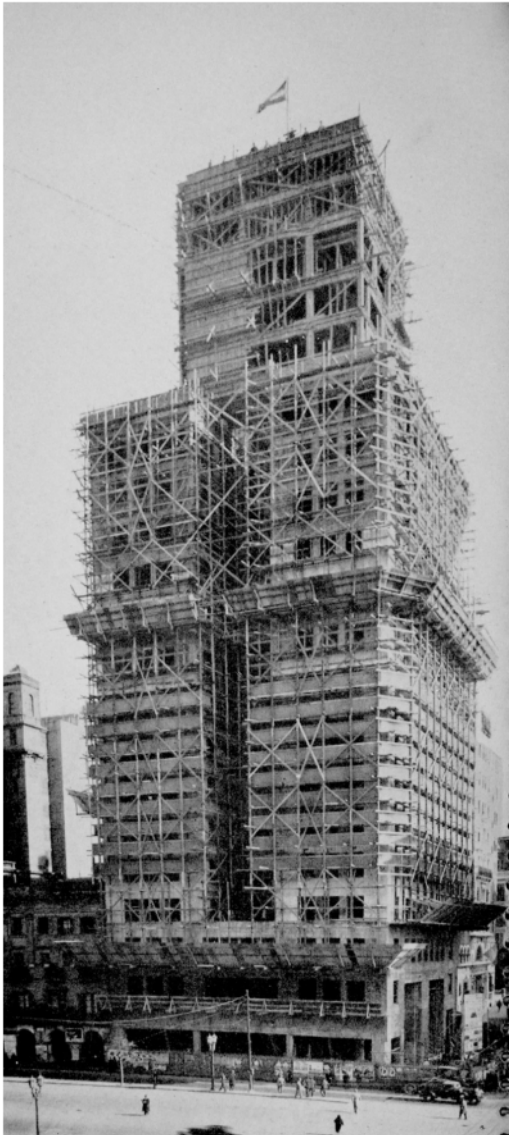
Figure 2. The COMEGA building under construction. (source: GEOPÉ 1938).
