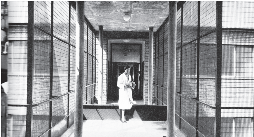
Figure 11.2 Entry to animal rooms was only possible from a perimeter open-air corridor (fine netting prevented wild animals and birds from gaining entry to the corridor). Strategically placed material barriers allowed human movement whilst preventing undesired rodent movements
