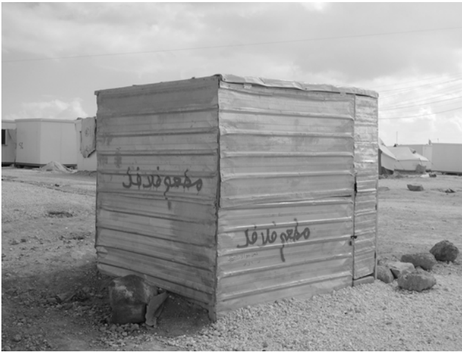
A falafel kiosk constructed entirely with zinco
