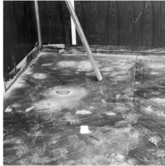
Wooden panels (Film faced plywood)
