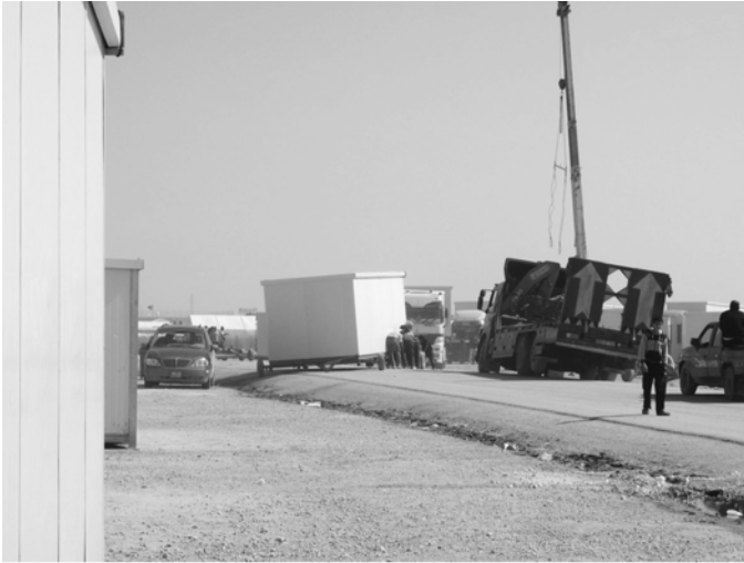
Refugees using a caravan conveyor to relocate a caravan after it had been placed on site
