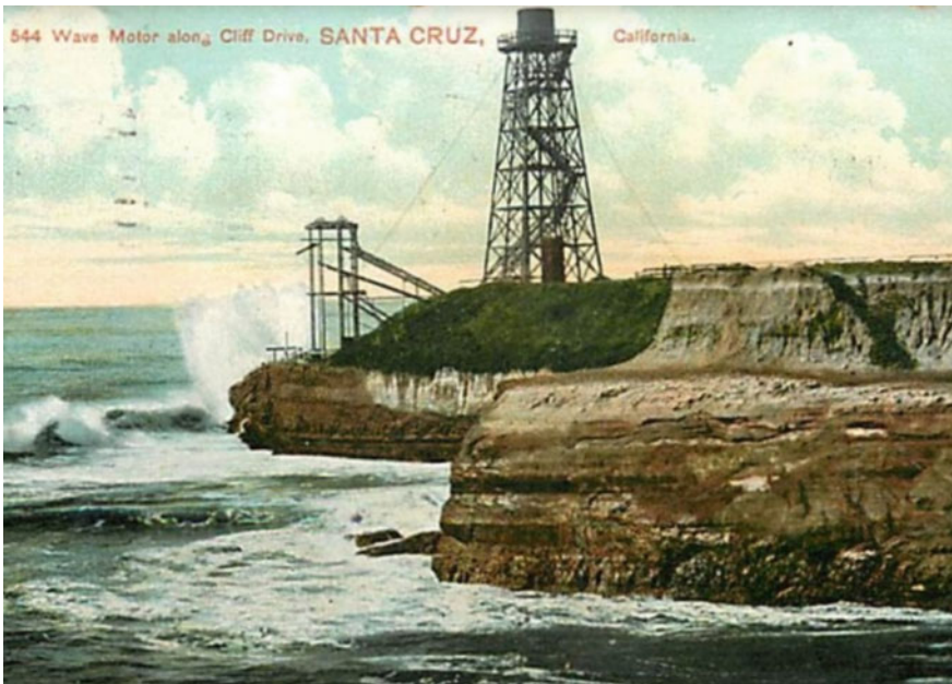
Fig. 2.4 Postcard from a “wave motor” experiment off the coast of Santa Cruz from 1898 [23]
