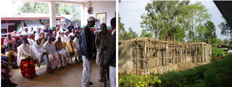
Figure 2: Nekemte Eye Clinic: Outpatient area and bed house under construction
