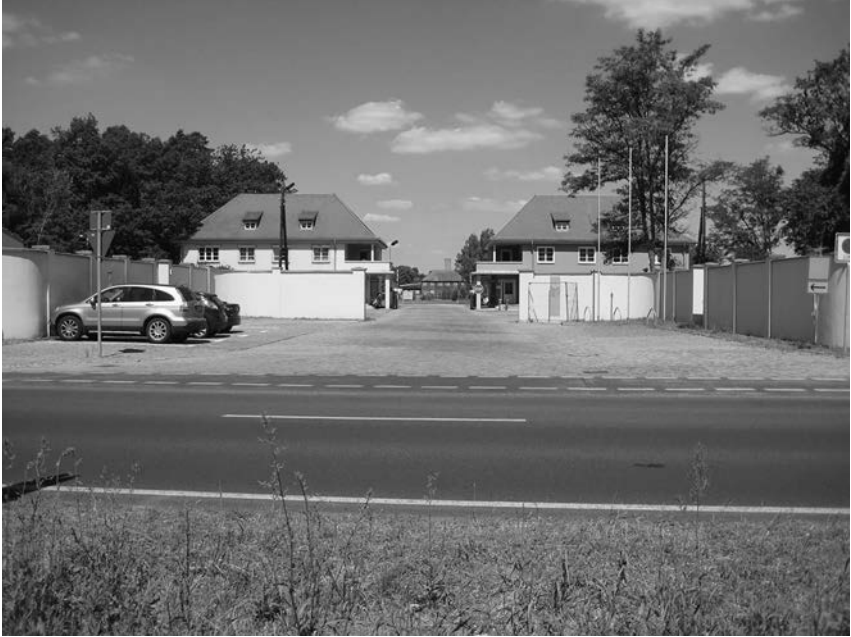
Figure 17. Police Academy of Brandenburg, entrance gate on Bernauer Straße 146, Oranienburg (2010). © Daniela Sandler
