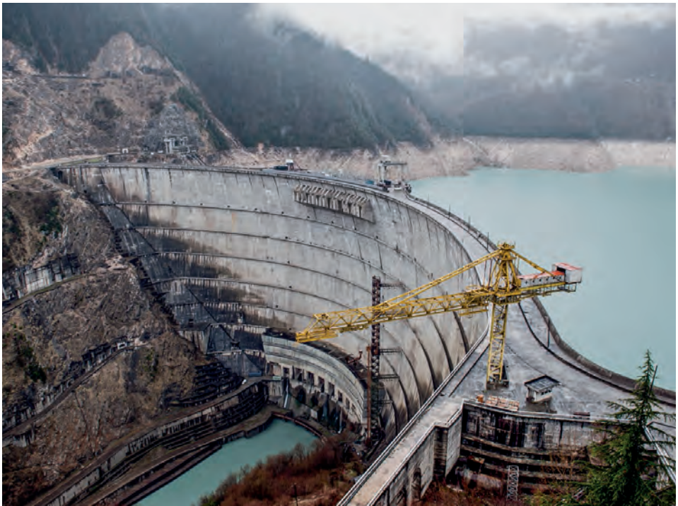
Since 1998 the EBRD has helped to restore and renovate Georgia's Enguri Dam, the world's second largest arch dam. © EBRD
