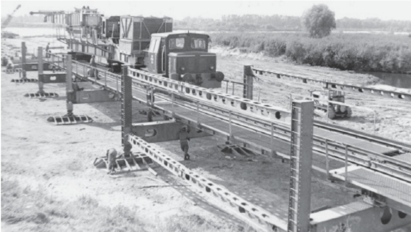
The assembly of a REM-500 overpass during the VISTULA 75 exercise. An SM03 locomotive from the Ammunition Depot in Stawy near Dęblin in the foreground, photo by Colonel J. Jarzyna (courtesy of Colonel J. Jarzyna)
