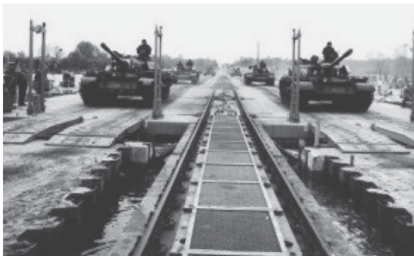
A modern road-rail crossing constructed in Wysokie Koło with the use of BP-150 barges during the VISTULA 75 exercise (courtesy of Colonel J. Jarzyna)
