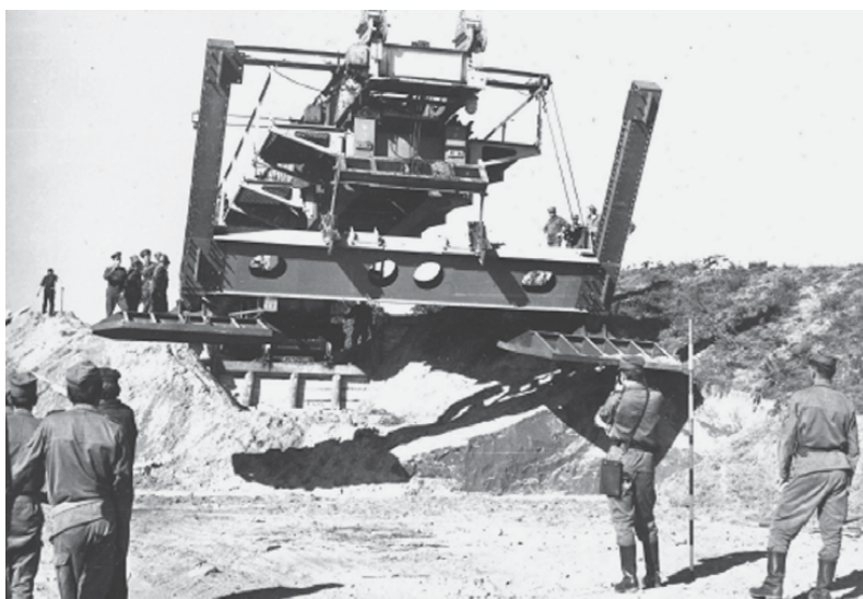
The assembly of a REM-500 overpass during the preparations for the VISTULA 75 exercise, photo by Colonel J. Jarzyna (photo courtesy Colonel J. Jarzyna). The required exercise uniform included a mandatory helmet, weapon, and a gas mask.
