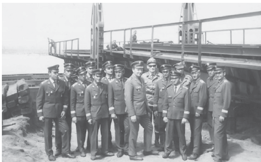
The Nowy Dwór near Kwidzyn crossing, 1969. A platoon of ensign cadets of the Officers' Military Engineering Academy in Wrocław, adjustable NZM-56 bridge support connected to the ferry via NZM-56 park structure components in the background (photo courtesy of Colonel Józef Sz wajka)
