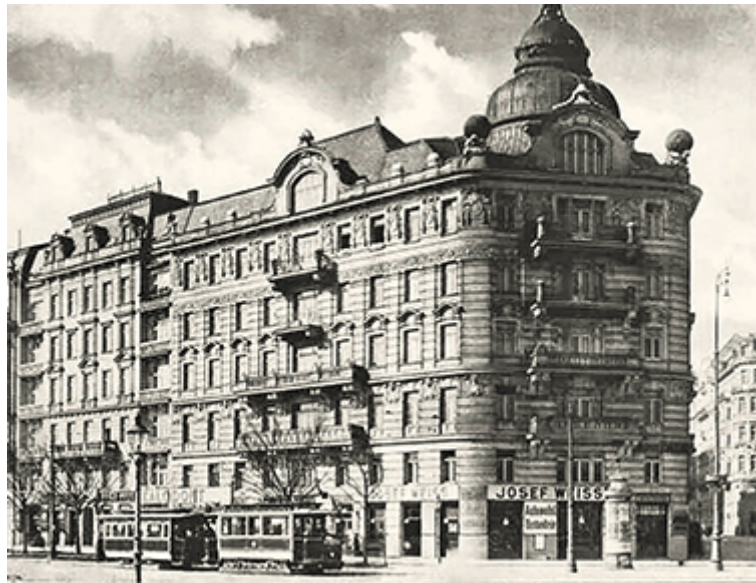
16. Jakob Gartner , apartment house, Vienna 1, Stubenring no. 2, built 1905/ Wiener Bauindustriezeitung 1907
