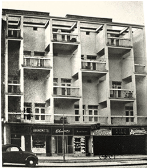
95. Egon Riss , apartment building, Vienna 19, Heiligenstädterstr. no. 95, built 1936 / Österreichische Kunst 1938
