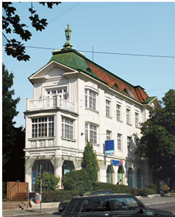
41. Julius Wohlmut , Grinzinger commercial building, Vienna 19, Allee no. 1, built 1913 / Prokop
