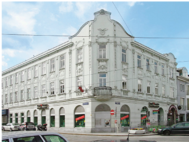
51. Neumann Tropp , apartment building and office building of the Zahnradbahn , Vienna 19, Nußdorfer Platz no. 5 / Prokop
