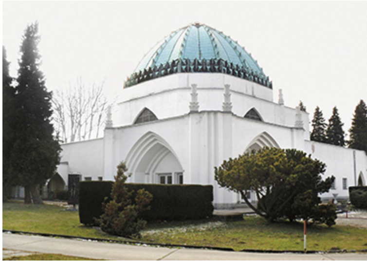
46. Ignaz Reiser , entrance hall to the new Jewish section of the Zentralfriedhof, Vienna 11, built 1928 (partly preserved) / Prokop
