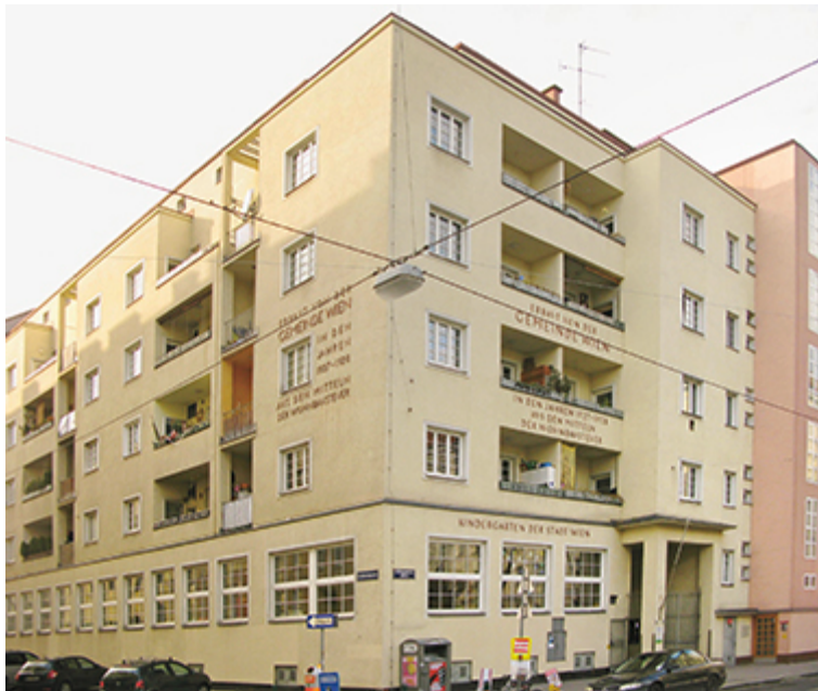
64. Walter Sobotka , municipal housing development, Vienna 3, Schrottgasse nos.10–12, built 1927 / Prokop
