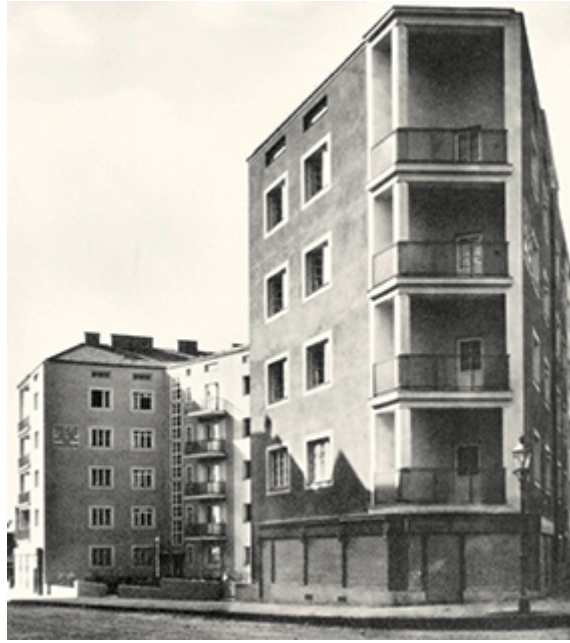
56. Josef Frank , housing development, Vienna 14, Sebastian-Kelch-Gasse nos. 1–3, built around 1928 / Moderne Bauformen
