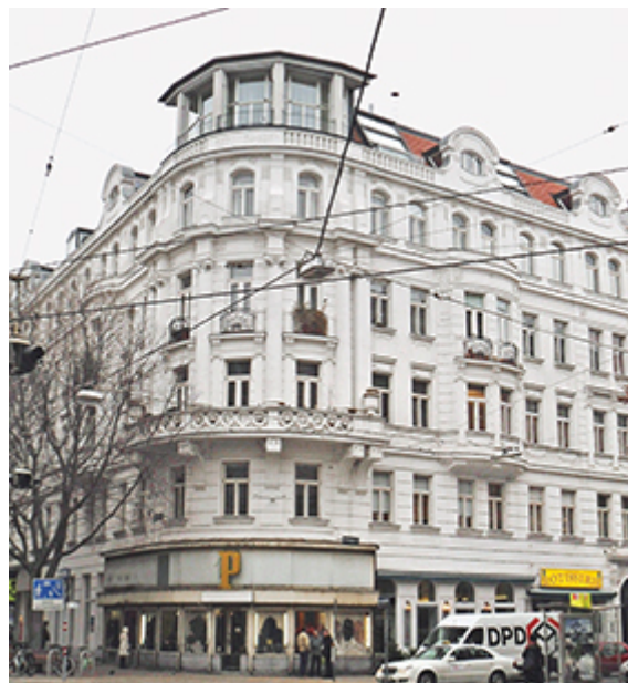
13. Jakob Modern , Servitenhof, Vienna 9, Berggasse no. 25, built 1904 / Prokop
