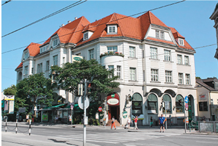
28. Arnold Karplus , apartment building, Vienna 14, Nisselgasse no.1, built 1912 / Kulturgut
