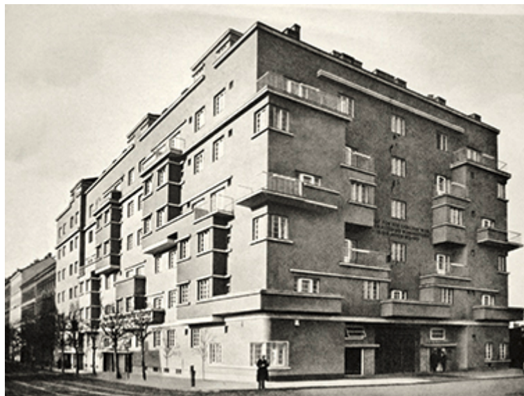
77. Josef Berger & Martin Ziegler , municipal housing development, Vienna 3, Schlachthausgasse nos. 2–6, built 1926 / Moderne Bauformen
