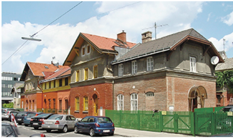
4. Josef Unger , workers' housing, Vienna 10, Kiesewettergasse 3–15, built around 1886 / Prokop
