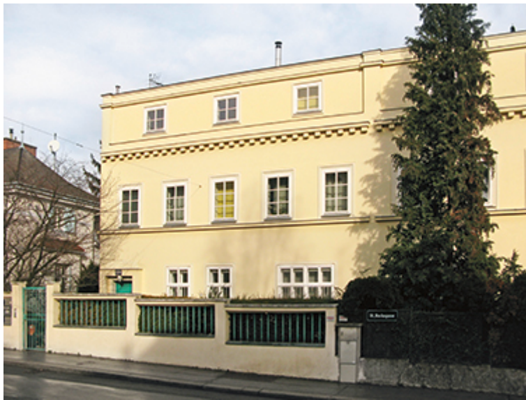
114. Erich Ziffer , pair of houses, Vienna 18, Hockegasse no. 88, built 1924 / Prokop
