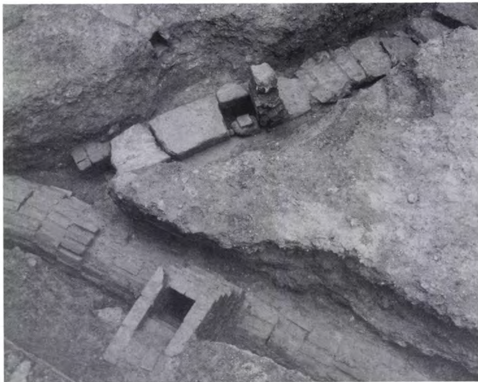
b. Brick culvert, F118, in the east wing, with a drain leading into it.
