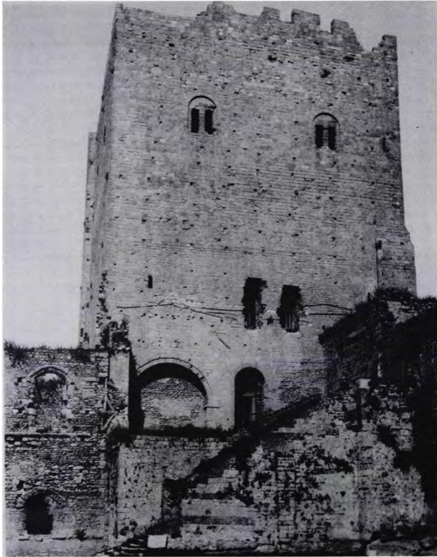
a. The east side of the keep c. 1930 showing the stairs against the outer wall of the forebuilding which were removed as part of the renovations.
