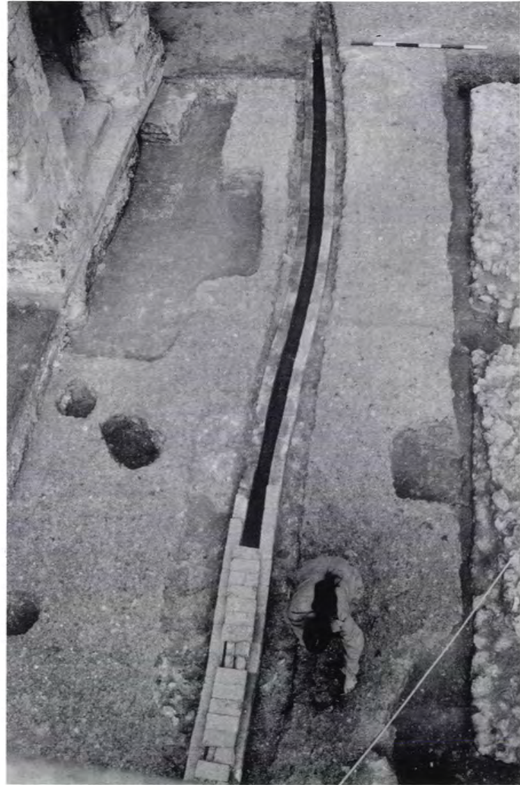
b. Brick culvert, F101, running across the inner bailey courtyard.
