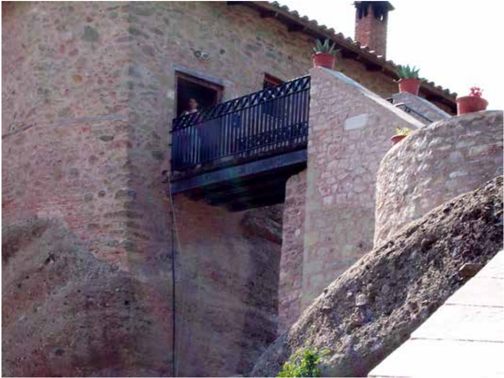
Figure 30: The Roussanou monastery's access bridge after restoration (source: author's photo).
