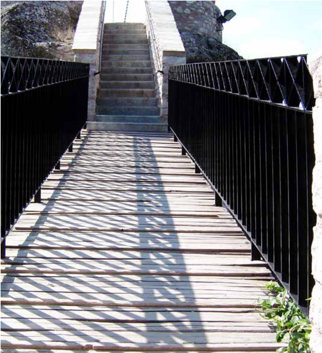
Figure 31: The Roussanou monastery's access bridge after restoration: detail (source: author's photo).
