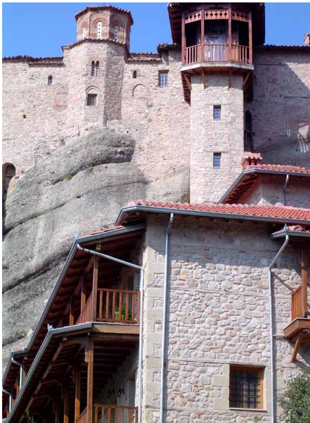
Figure 33: The Roussanou monastery: the tower-lift connecting the five storey building with the original monastery (source: author's photo). The tower-lift ends on its top to a roofed structure that looks like a balcony of the original monastery.
