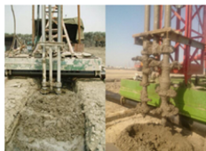
Figure 1. JBS-II biaxial mixing drilling system.
