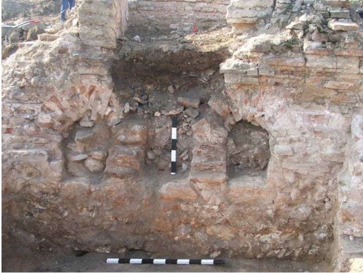
Fig. 3: Late antique thermae – detail of the suspensura in the room Nr. 1 (Photo: Z. Dimitrov).
