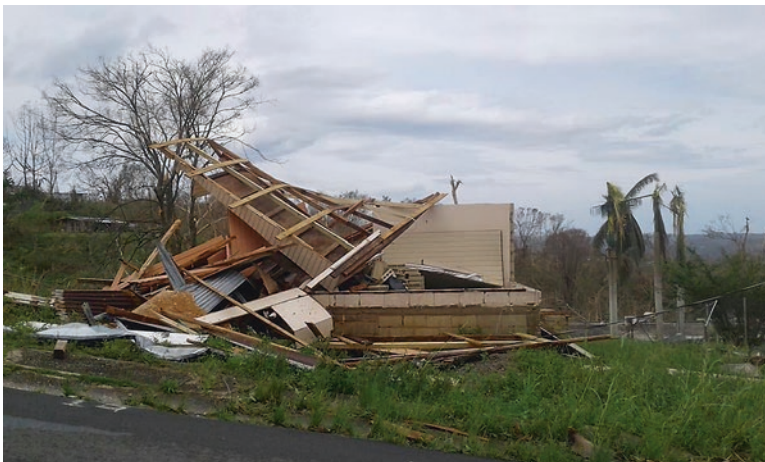
Fig. 6.1 House shattered by the hurricane winds
